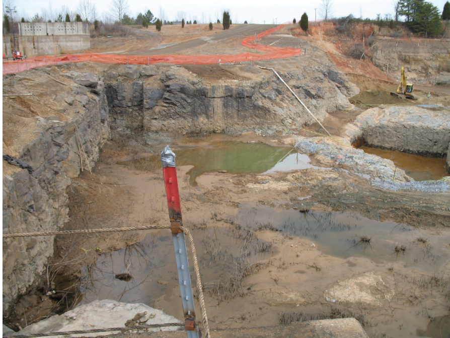
Post draining excavation condition prior to cleaning. Sediment and water covered foundation surface in former CNS Unit 2. View towards north, March 3, 2006.
