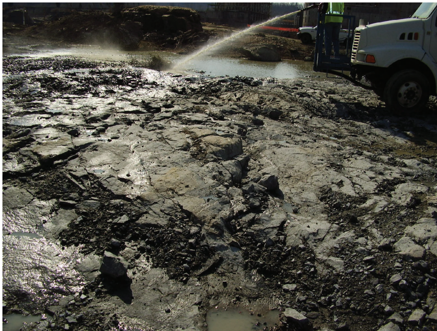
Example of rock cleaning. Water spray is used to remove excessive sediment from exposed rock surface. View towards west, March 3, 2006.
