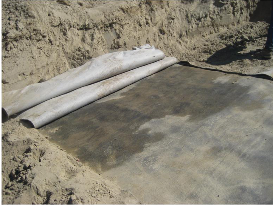
Fig. M. 3. Minimal moisture observed at GDL-GM interface upon exposure.
