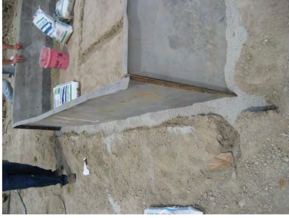
Fig. A.11. Cover soil removed prior to SDRI installation.
