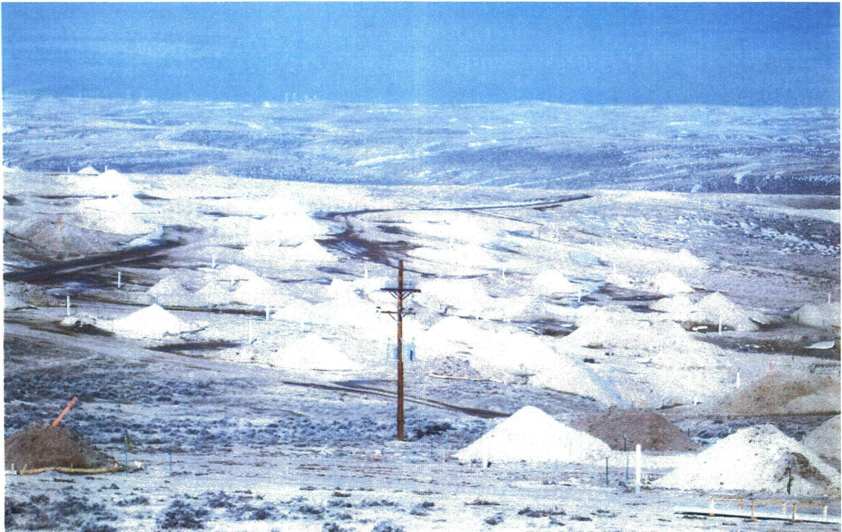
Figure 2 MU-10 wellfield development; topsoil stockpiles placed away from drilling activities and clearly marked, routes for vehicle use are clear, areas without disturbance can be identified, sediment control placed around stockpiles
