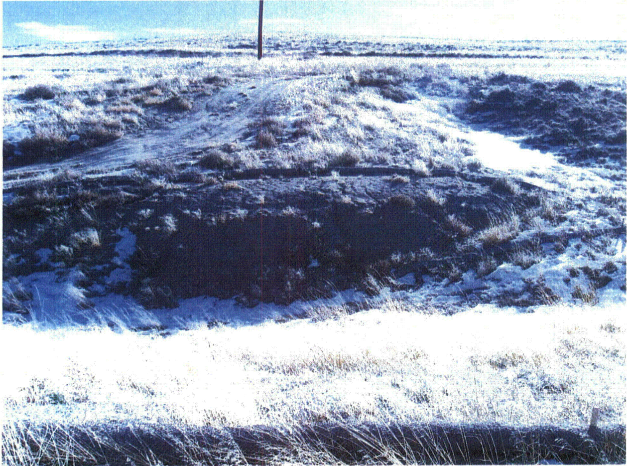
Figure 1 South slope of drainage in MU-9; straw waddles used to control sedimentation; steep slope without vegetation likely to continue to erode
