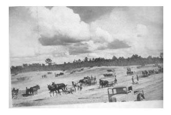
Excavation procedures were a remarkable mix of modern technology and old-fashioned muscle. "Working alongside the modern, powerful excavating machines were men loading trucks with shovels and mule teams dragging old-fashioned scrapers. Huge tractor-scrapers, draglines, belt conveyers, tractor-hauled wagons, and trucks all
