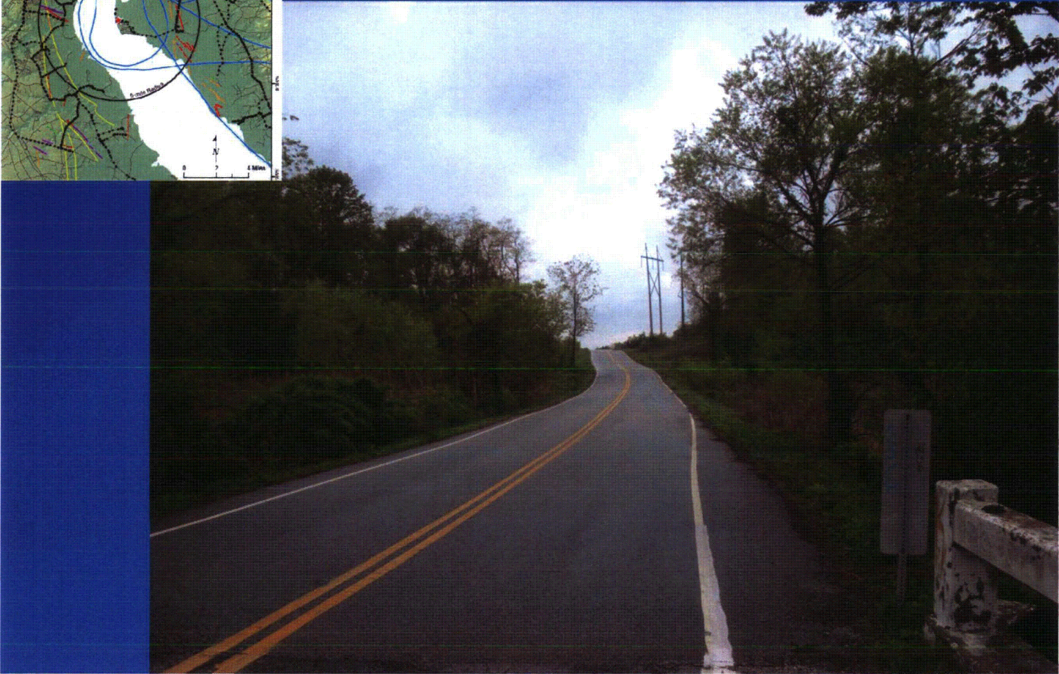
Figure RAI-44-4-3. View of Terrace Risers in Delaware.
