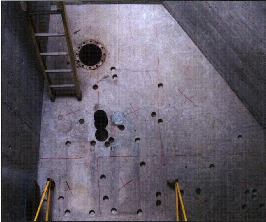
(NW Wall showing pipe penetrations, remediated concrete and ledge)
