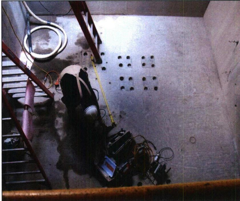
(West Wall showing concrete remediated around penetrations)
