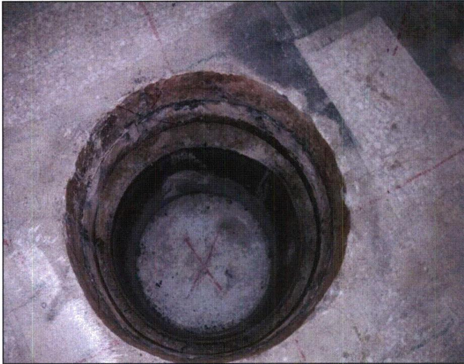
(irregular surface from core drilling to remove contaminated pipe in Room 4 Wall)
