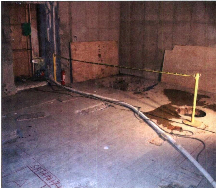
(grouted PCW piping entrance/exit from PPH inside sheath below Room 4 floor)
