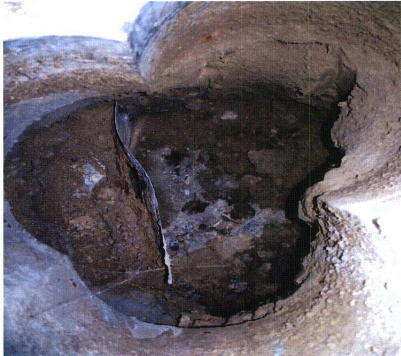
(penetration in Room 3 ceiling showing rough edges and rebar)
