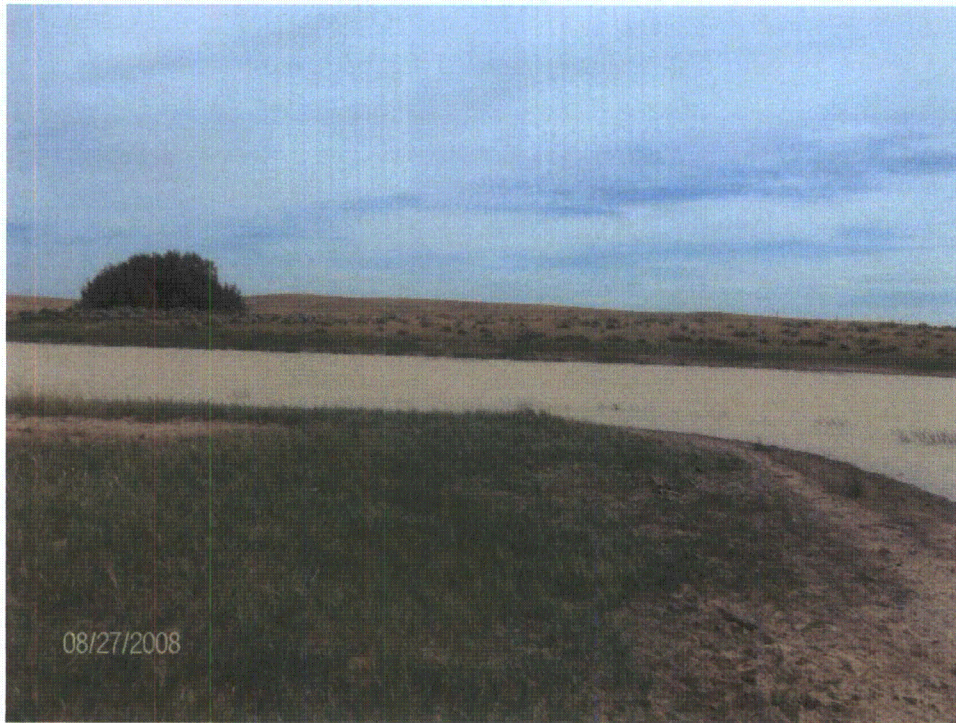
Photo 35: Downstream from U18
