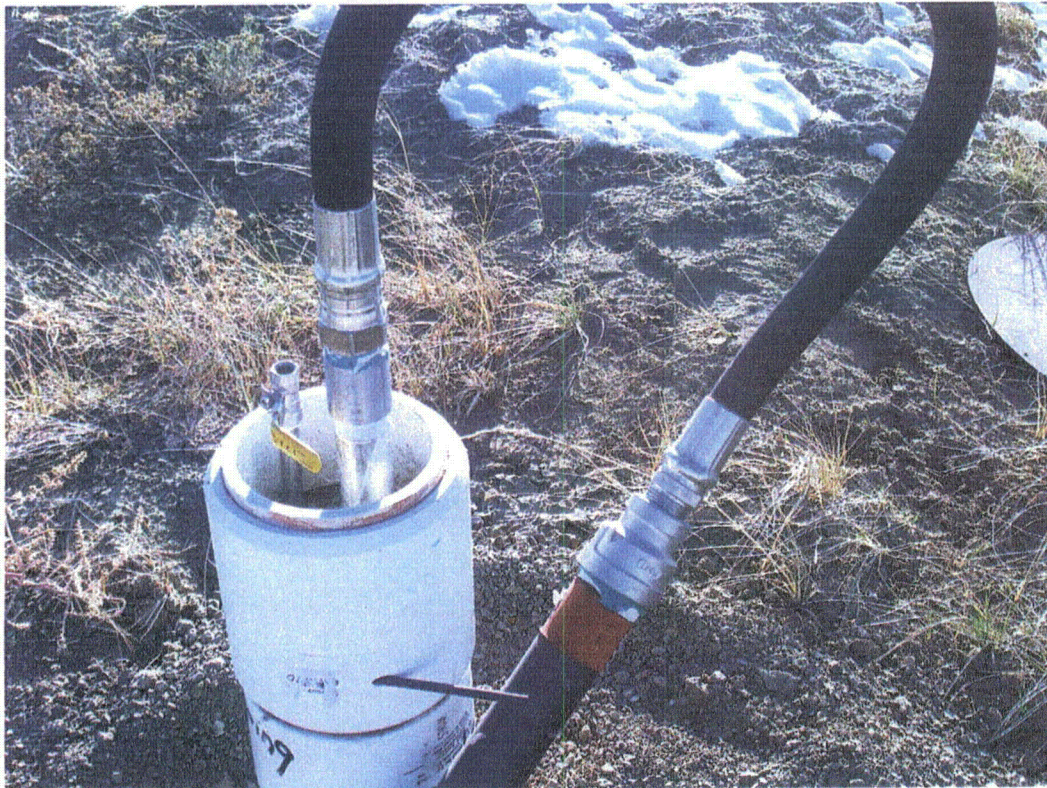
Figure 2 Replaced cracked coupling at EI-287A
