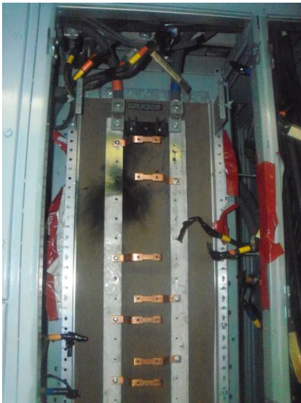
FIGURE 8 - DC DISTRIBUTION PANEL D11-2 INSPECTION AND REPAIR SEVERAL DAYS AFTER THE EVENT
