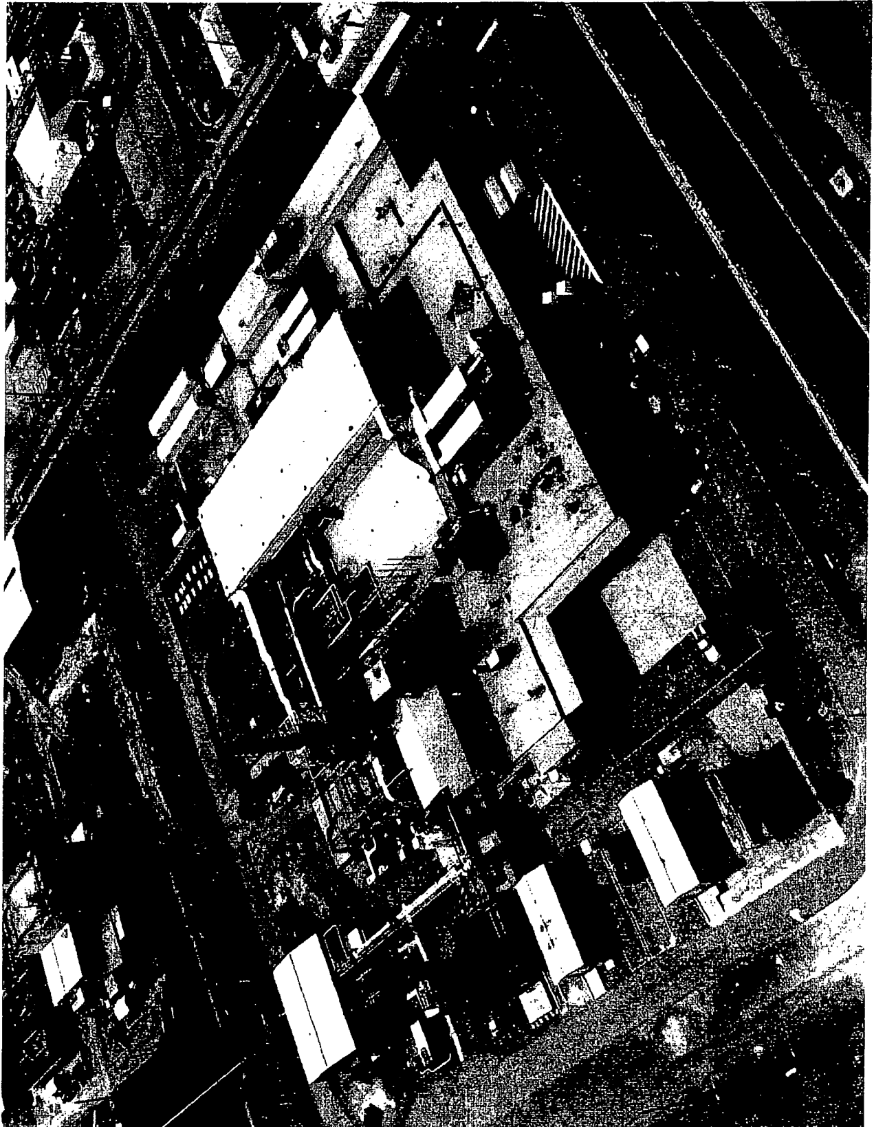
Figure 1.2-7 Naval Fuel Facility Aerial View
