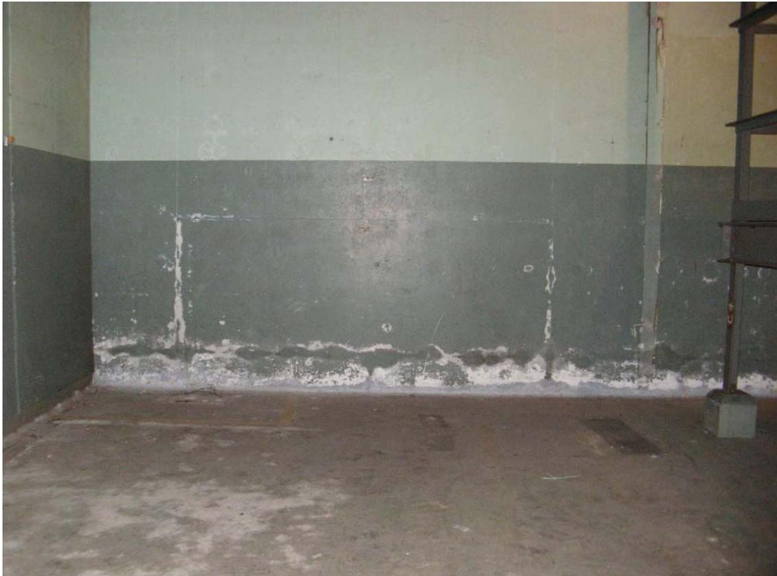
Figure 6.2 Efflorescence in R-reactor Assembly area [19].
