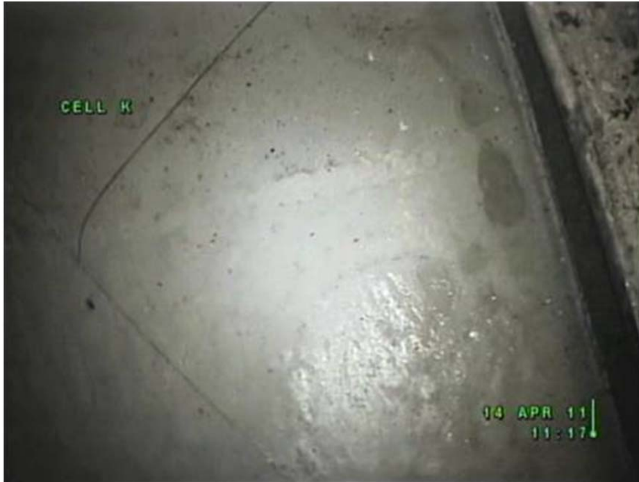
Figure 3.2-4: Cell K, West Wall Grout Surface
