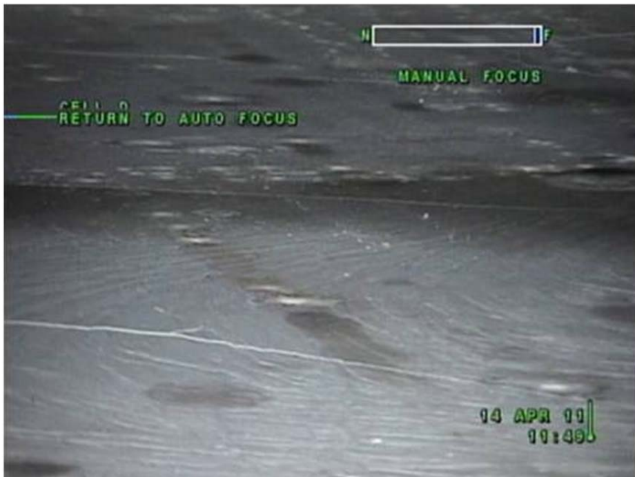
Figure 3.2-5: Cell D, Grout Surface
