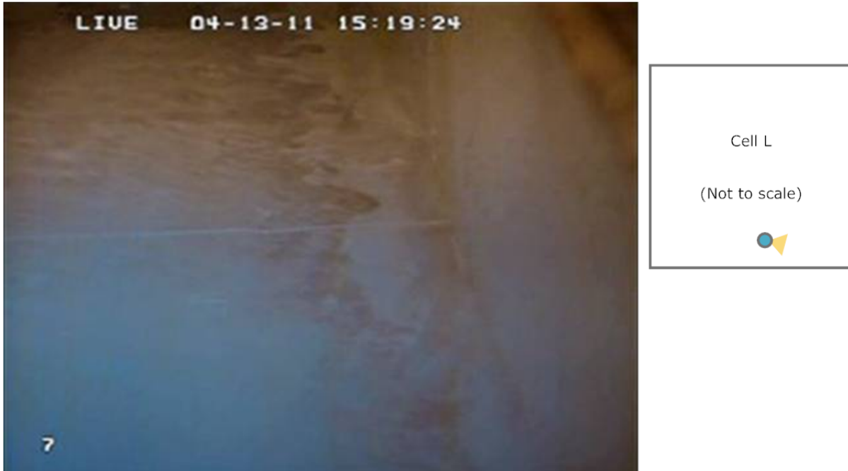
Figure 3.2-8: Cell L, Grout Surface
