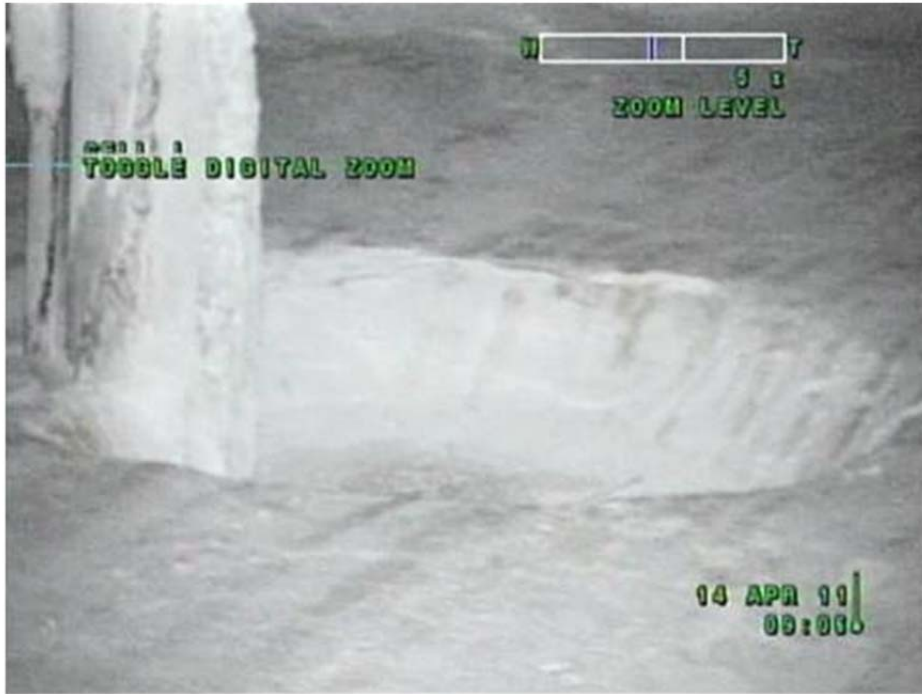
Figure 3.3-1: Cell I, Grout Surface Variation
