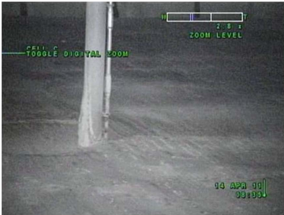
Figure 3.3-2: Cell C, Grout Surface Level
