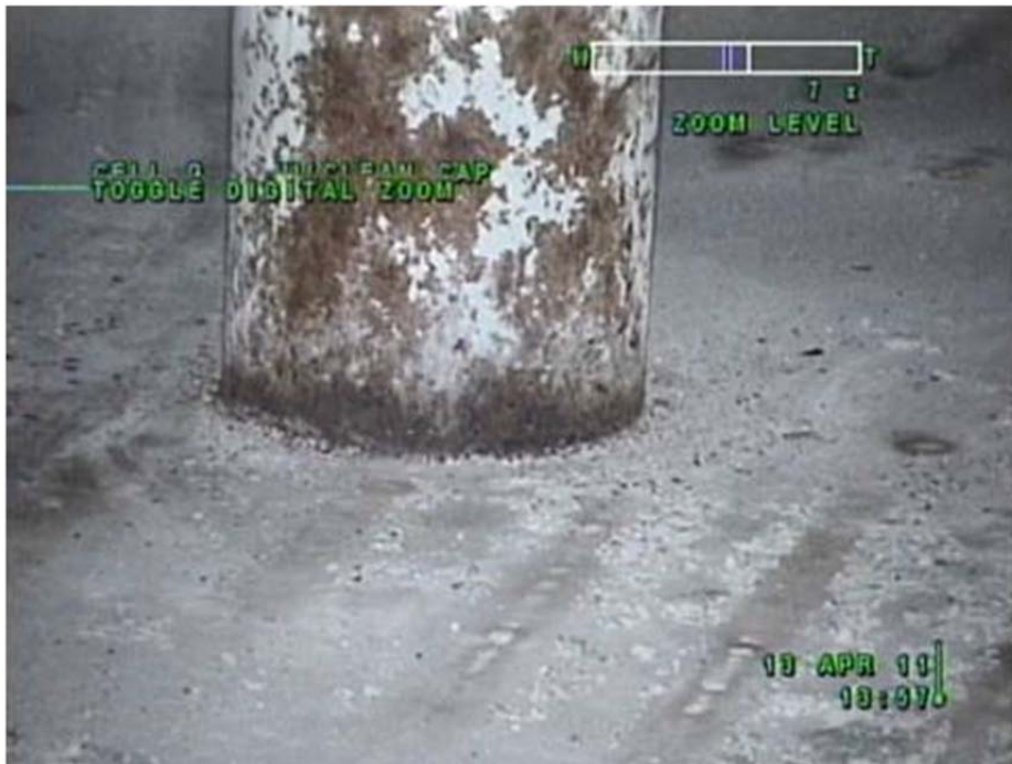
Figure 3.1-2: Cell G, Column-Grout Interface
