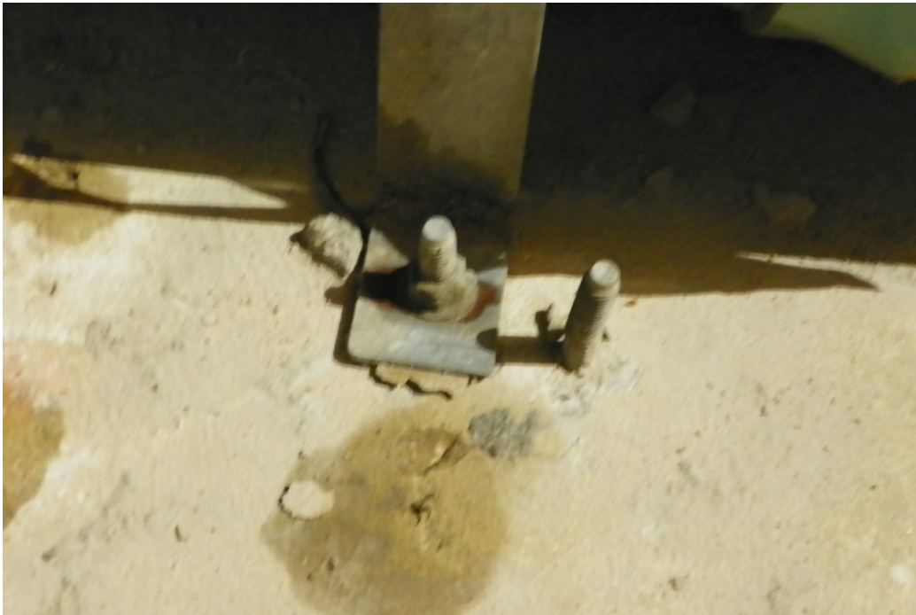
Figure 1.5-3: Typical Vault 4 Anchor Bolt Installation – No Cracking or Voids
