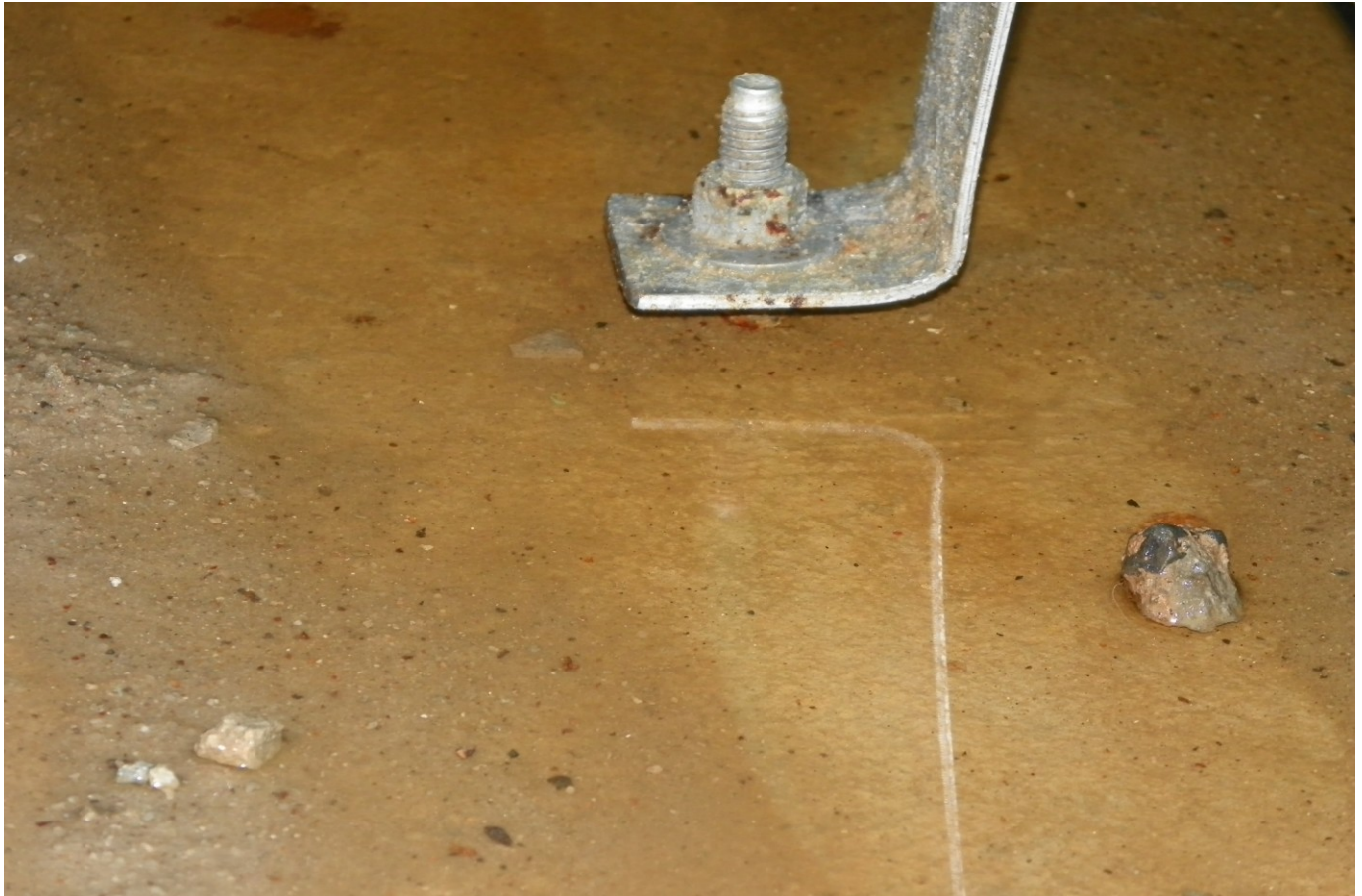
Figure 1.5-4: Typical Vault 4 Anchor Bolt Installation – In Freestanding Water
