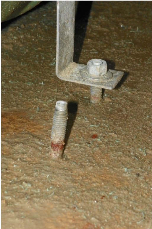
Figure 1.5-1: Typical Vault 4 Anchor Bolt Installations – Used and Unused
