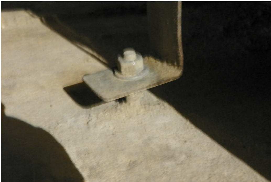
Figure 1.5-3: Typical Vault 4 Anchor Bolt Installation – No Cracking or Voids
