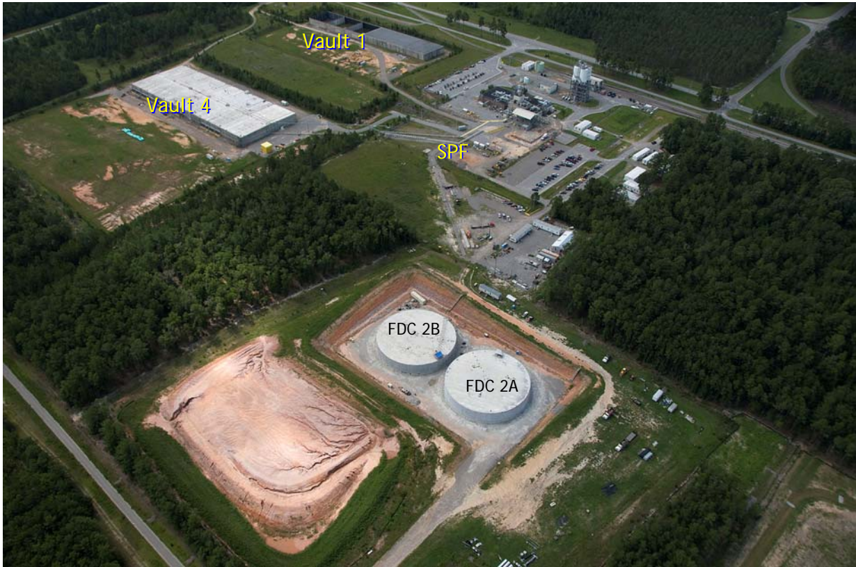
Figure 3.1-1: Saltstone Facility Aerial View
