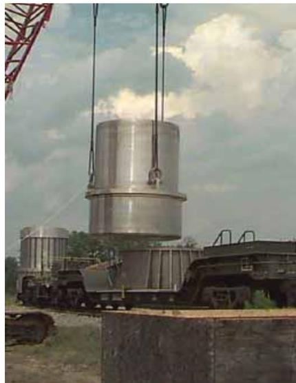
Figure 18. (Top) Photo showing partially covered naval reactor components of various sizes. Earth and a clay cap will be mounded over naval reactor waste prior to final disposal. There are two such facilities, the “old” (two top photos) and “new” (bottom photo) facilities. (Bottom) Naval reactor component before it is placed in the disposal area (WSRC 2008).
