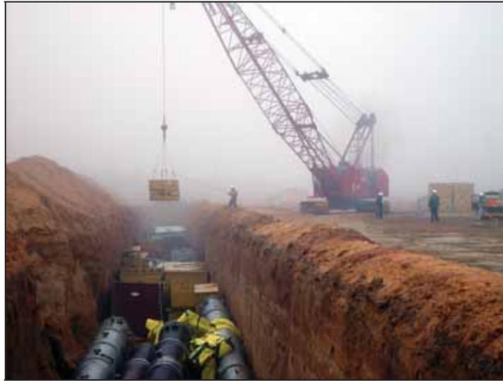
Figure 9. E-Area Slit Trench Facility showing a range of waste materials. Also note the red clayey sediment, characteristic of the upper sediment strata.
