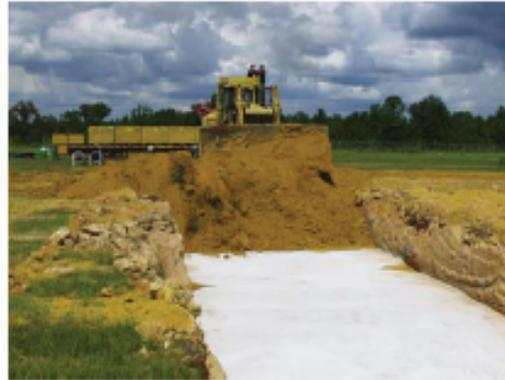
Figure 14. Sequence of steps in the disposing of waste as Components in Grout (CIG; WSRC 2008).
