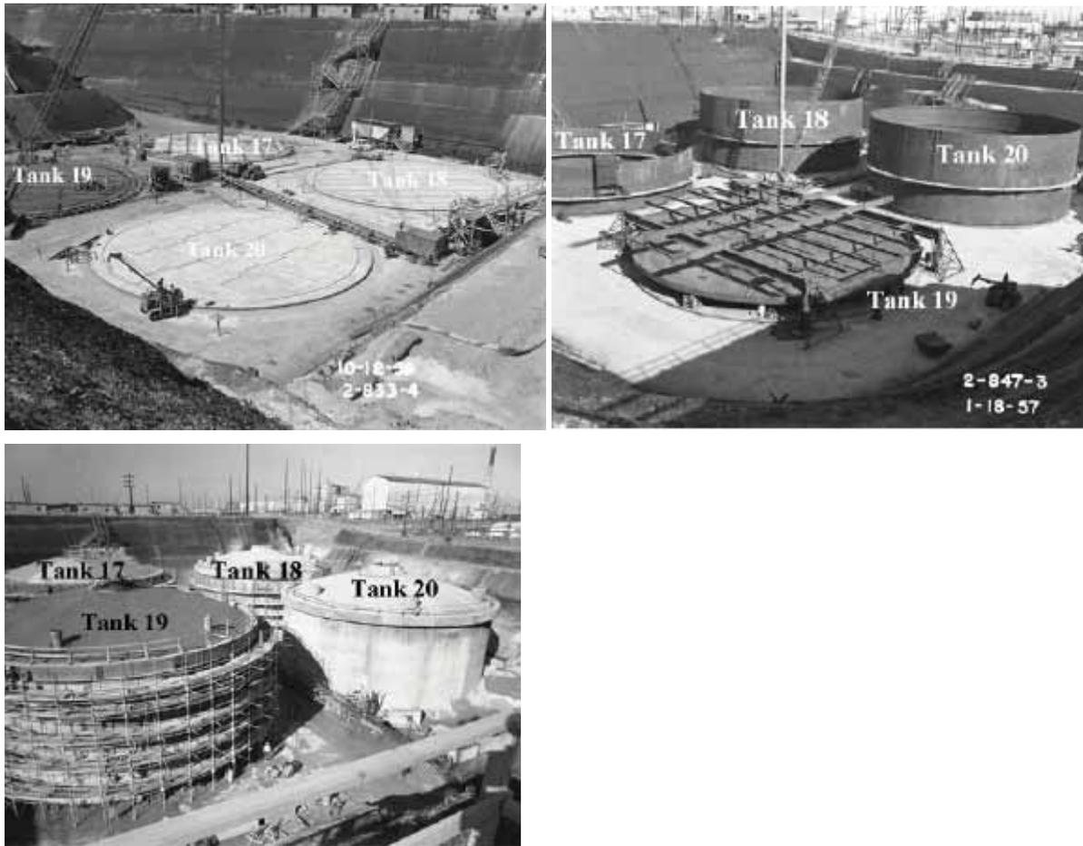
**Figure 23.** Examples of Radioactive Waste Tank construction. Top Left: 17-cm concrete basemat pads; Top Right: Carbon steel liners; Bottom Left: Tank concrete walls (note relative scale of tanks compared to men on scaffolding (photos from Buice et al. 2005).
