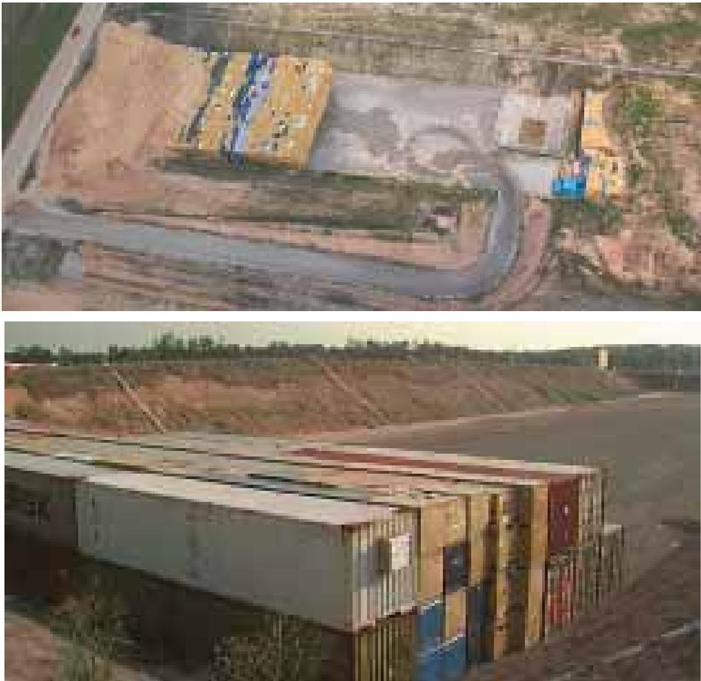
Figure 10. Engineered Trench: (top) aerial view and (bottom) close up of metal containers holding low level waste (WSRC 2008).
