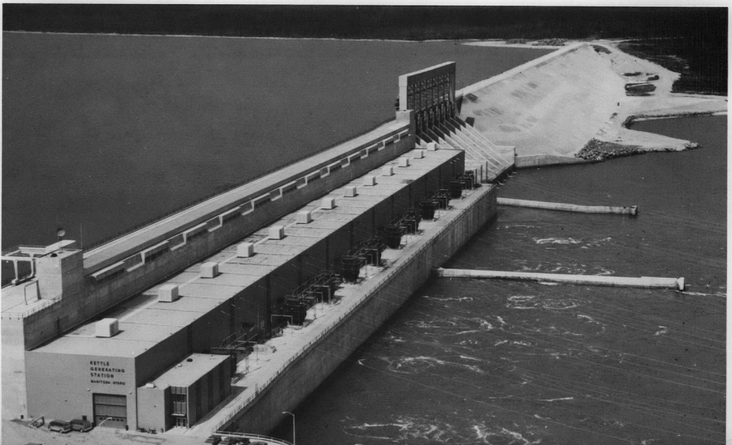
Manitoba Hydro Kettle Generating Station on Nelson River has 1,272 mw capacity.
