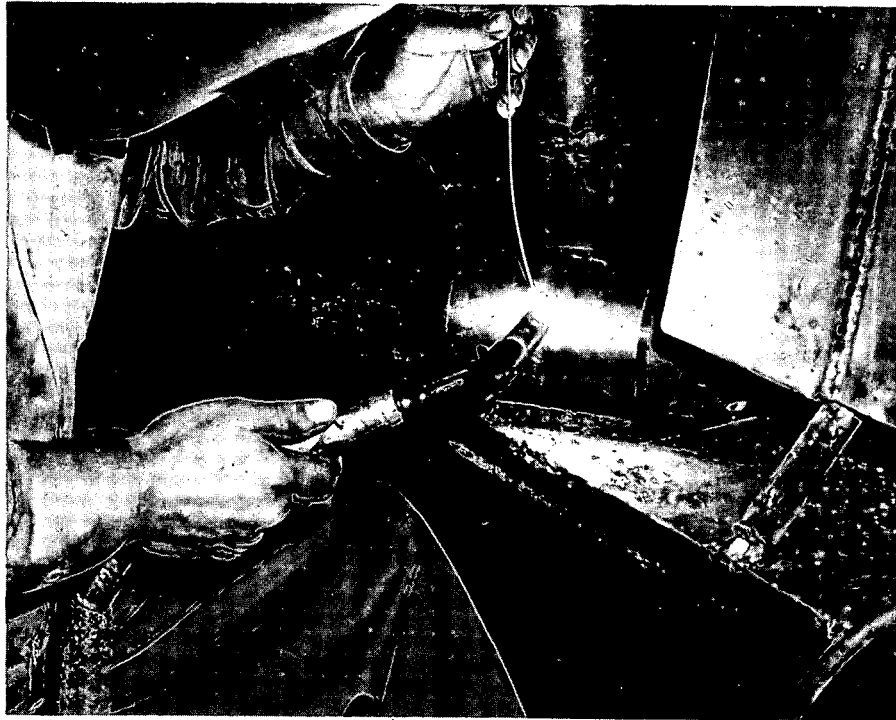
FIGURE E-17. TIG WELDING
