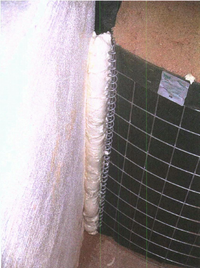
Figure 2-59. Expanded foam at abutment with concrete wall
