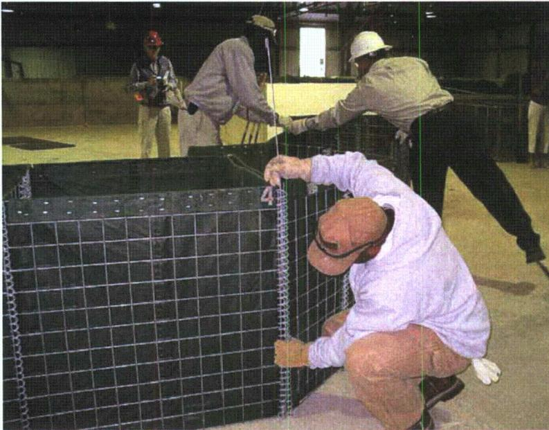
Figure 2-48. Pinning units together
