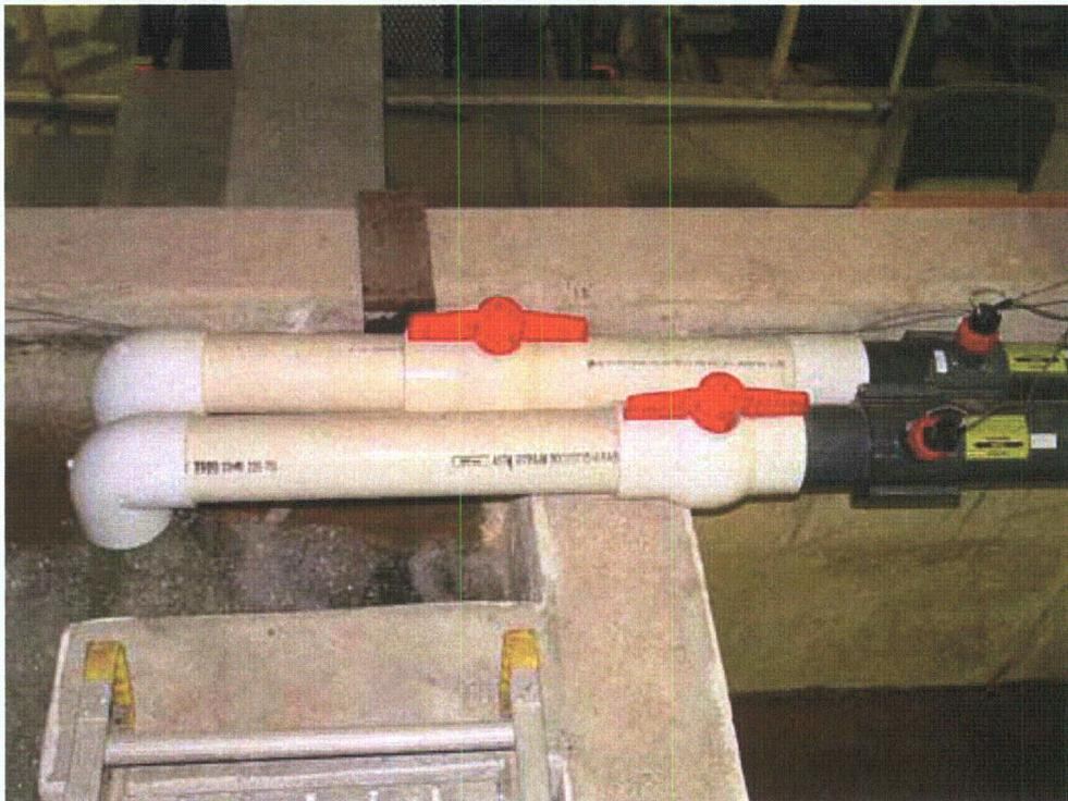
Figure 2-6. Sump pit outflow pipes and flow meters
