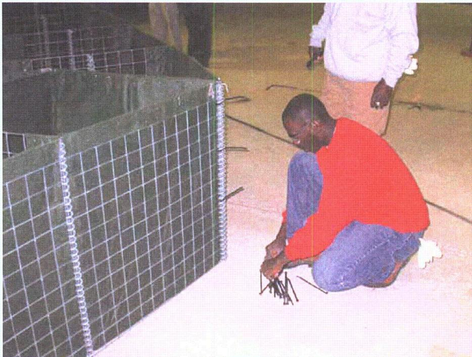
Figure 2-50. Cable ties at joint connections
