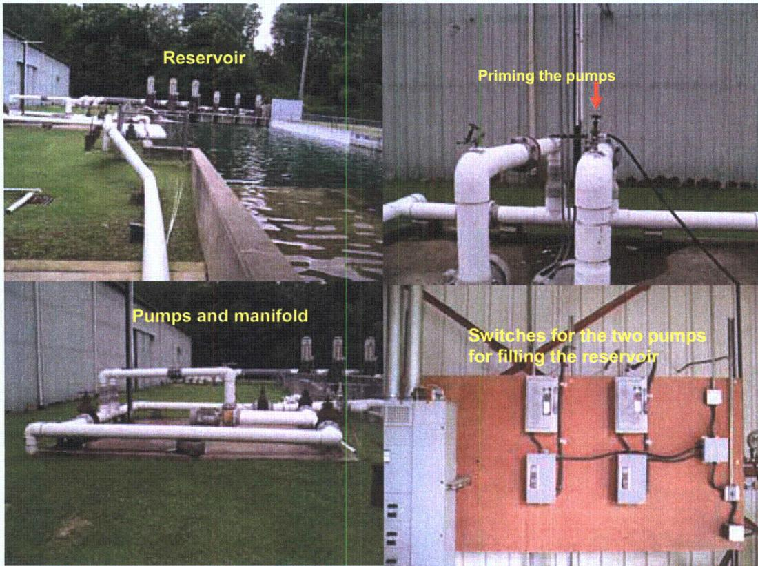
Figure 2-10. Reservoir-filling system
