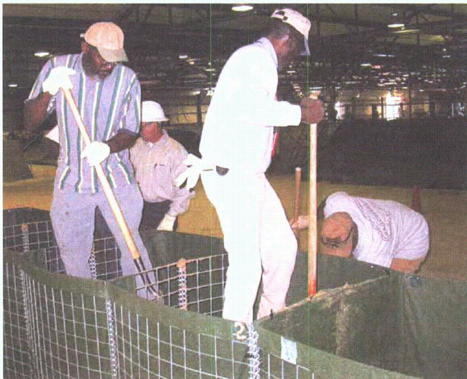
Figure 2-55. Leveling and compacting sand within each unit
