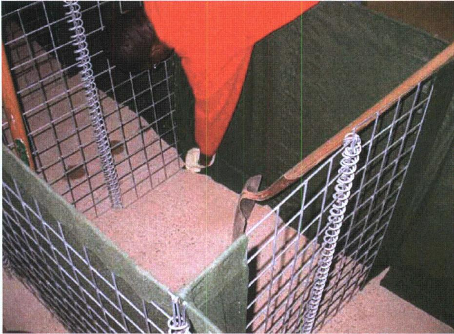
Figure 2-52. Securing flaps against concrete floor. Note center coils which are prefastened at factory
