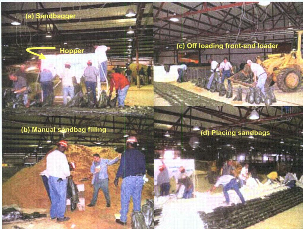
Figure 2-19. Sandbagging operation
