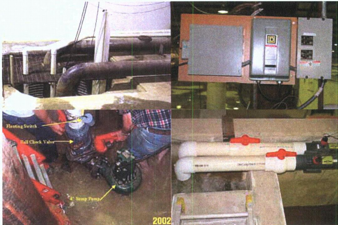
Figure 2-2. Sump pit containing two 4-in. pumps. Top left: top of sump pit. Top right: power control panel. Bottom left: 4-in. pumps in pit. Bottom right: 4-in. valves and flow meters
