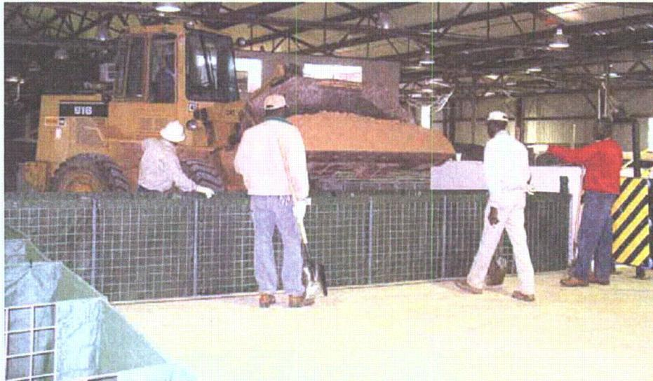
Figure 2-53. Filling with sand
