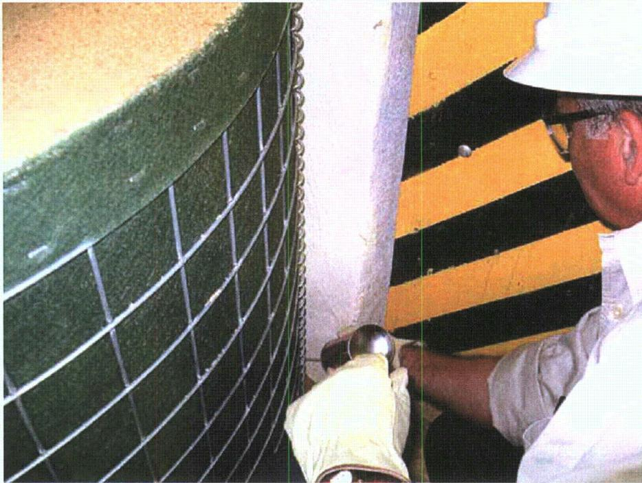
Figure 2-58. Sealing concrete wall abutment with aerosol foam
