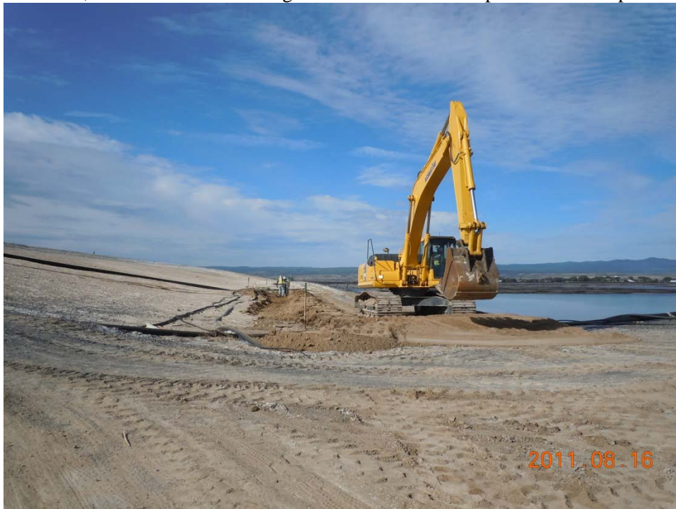
Initial construction of drainage ditch, looking South.
