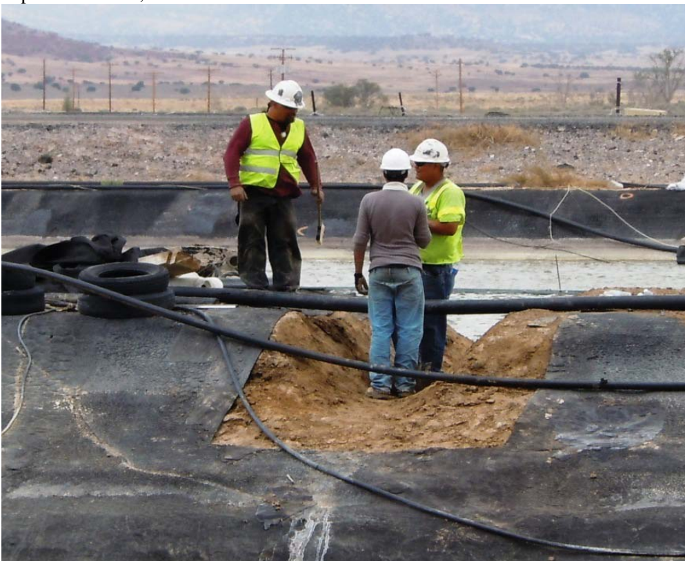
West – East Collection Ponds Cross-Ditch excavated for Liner Reconstruction
