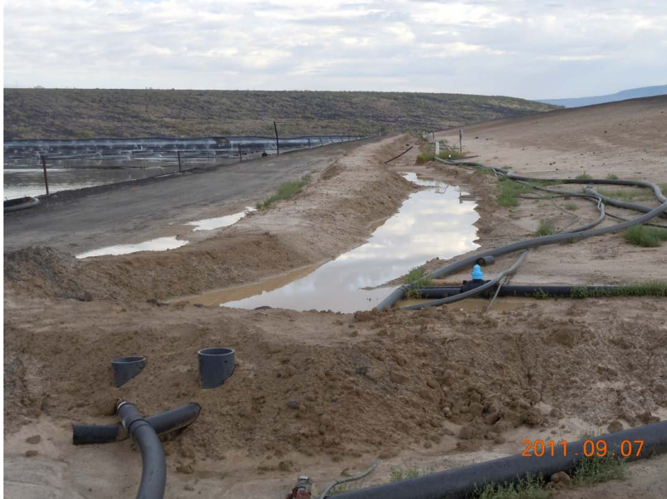
Completed drainage channel between Evap No. 1 and Evap No. 2, looking North.
