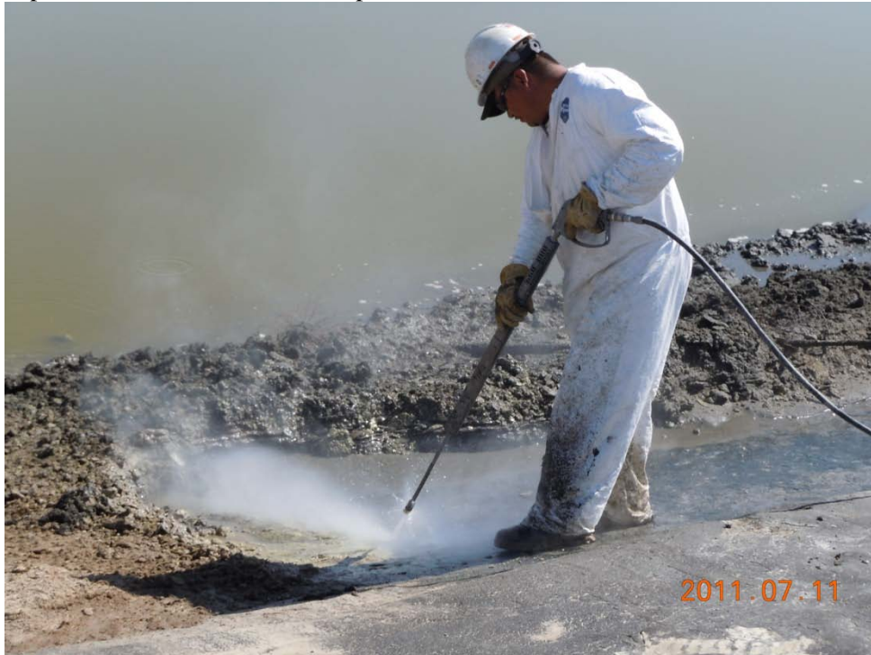
Evaporation Pond No. 1 SE Corner, washing sediment from liner with high pressure washer
