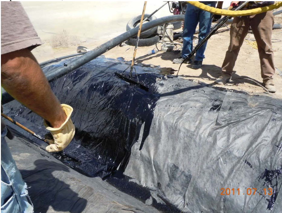
Application of Deery Oil over fabric
