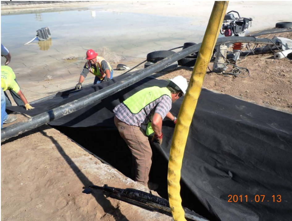
Installation of felt fabric material in Cross-Ditch
