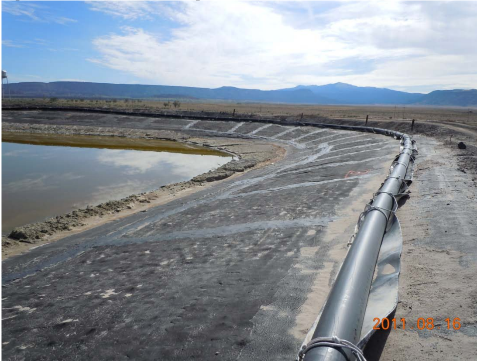
Deery Oil Liner System after repair. Note subbase recompact and seams sealed.
