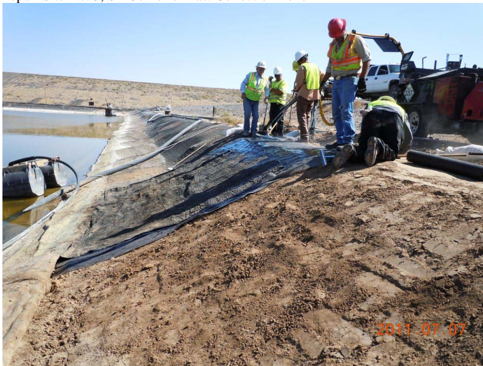
Reconstructed sub-base embankment, spreading of fabric and Deery Oil application
