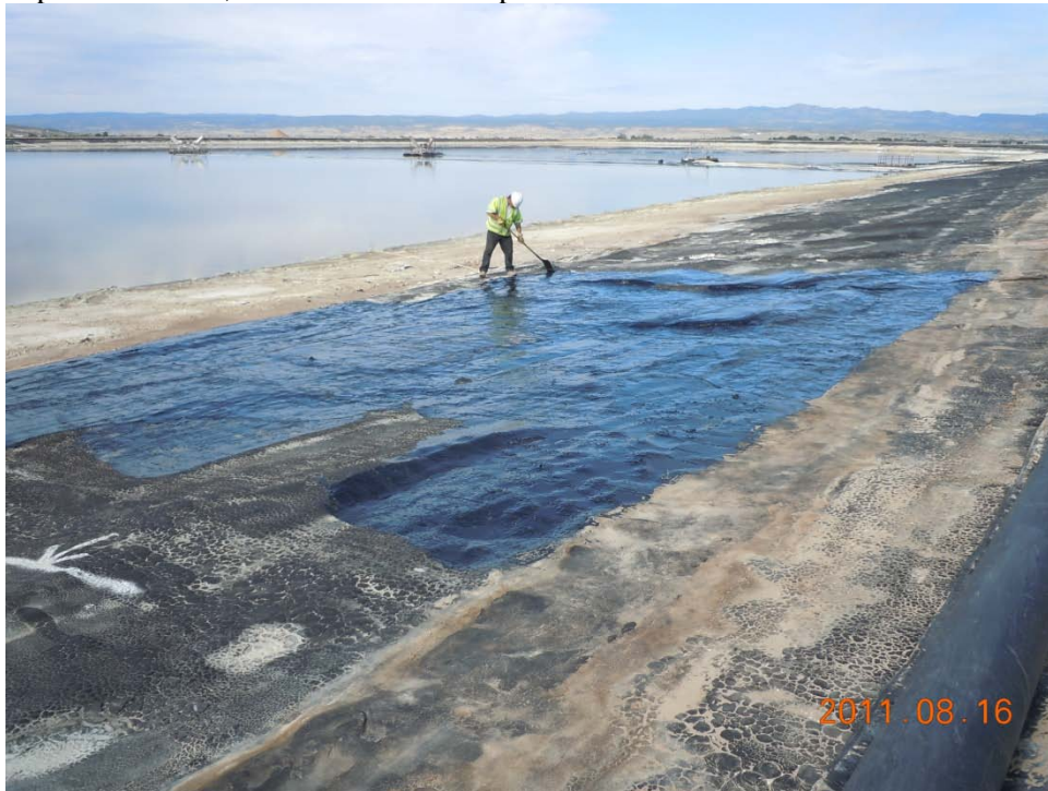
North embankment reapplication of Deery Oil top layer over weathered areas.
