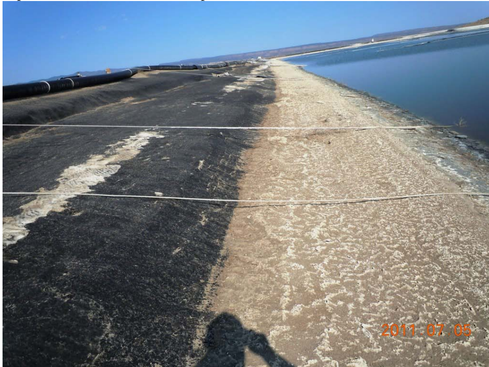
Evaporation Pond No. 1, SE Corner looking W. Pre-Existing Condition – wave benches
