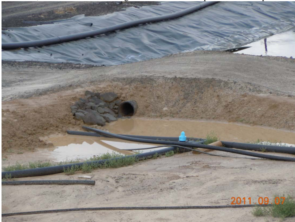
Completed drain pipe at South end of drainage channel, directing water into Evap No. 2
