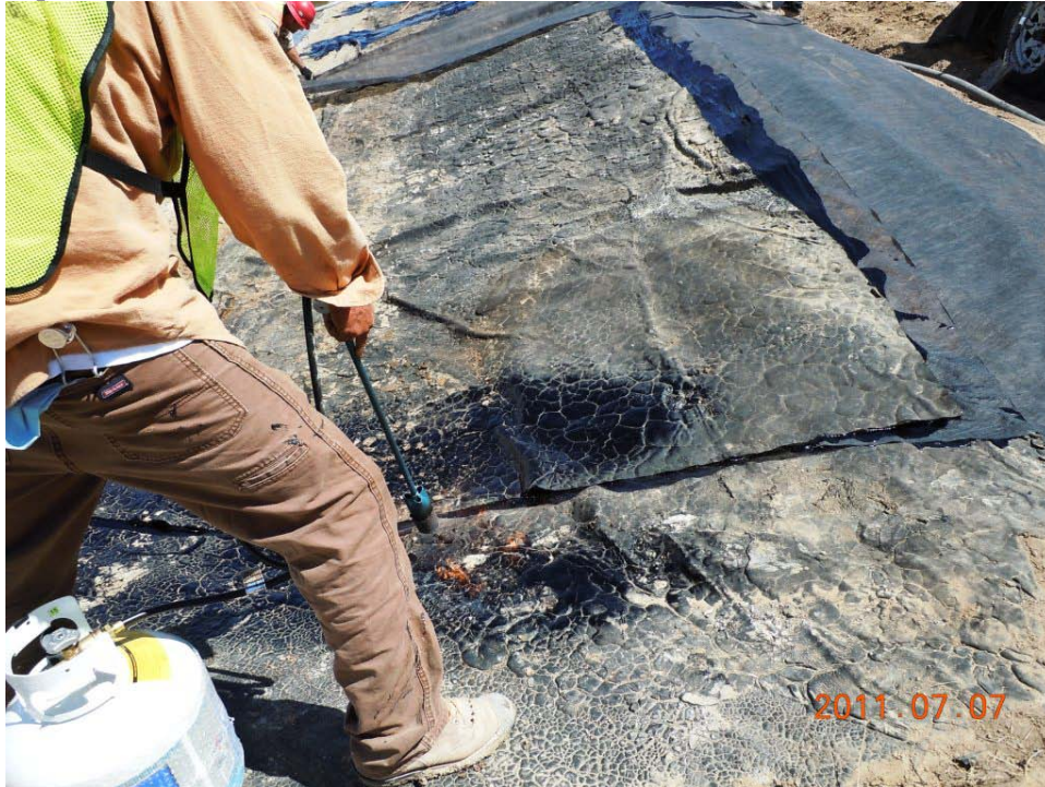
“Conditioning” of existing liner prior to fusion by Deery Oil liner system
