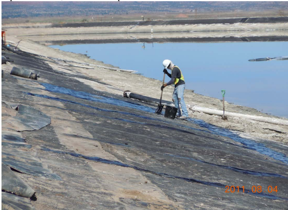
Applying Deery Oil to seams in liner after recompaction of subbase.
