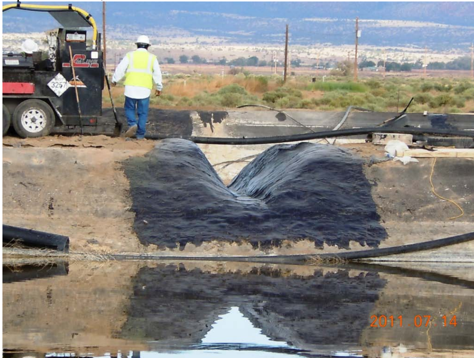
Completed Cross-Ditch between West and East Collection Ponds
