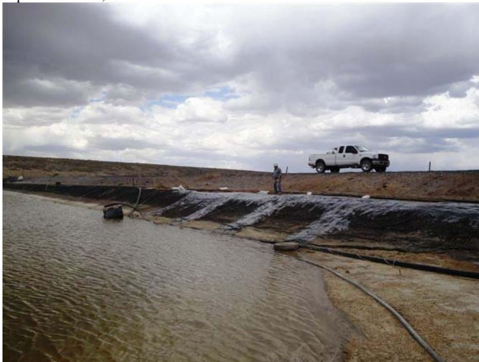
Deery Oil liner system repaired
