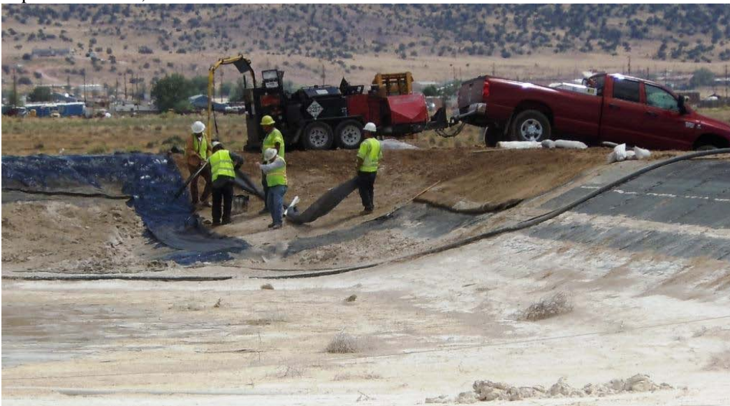
Reconstruction of Deery Oil Liner System in W Collection Pond SW Corner
