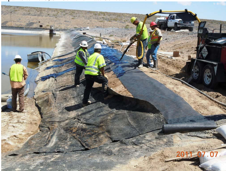
Adding additional liner to top of existing liner where top had been damaged
