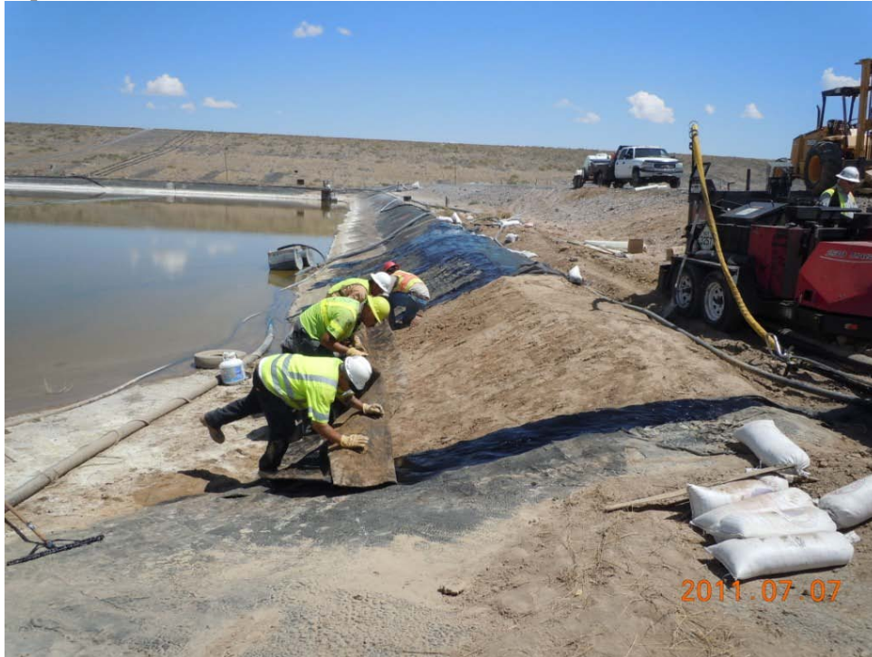
Rolling existing liner back into place for fusion with sides and top
