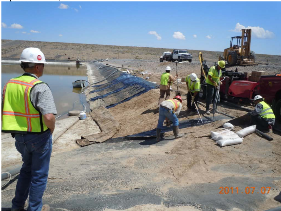
Fusion of section of existing liner system with fabric and Deery Oil & completed sections
