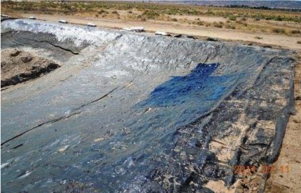
Reconstructed Deery Oil Liner System in W Collection Pond SW Corner
