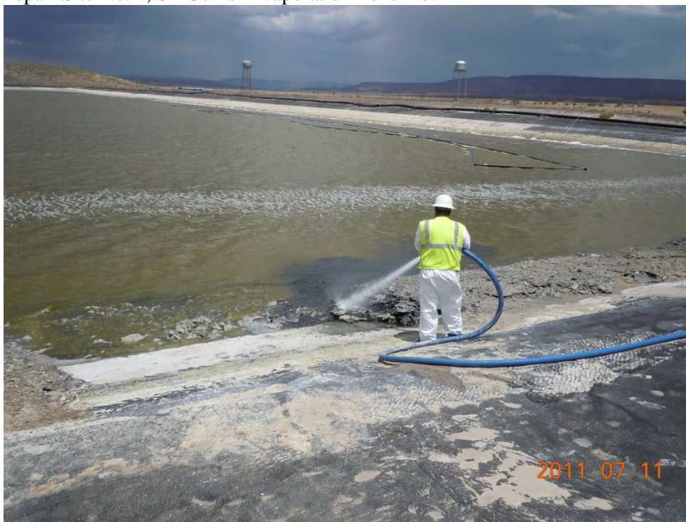
Evaporation Pond No. 1 SE Corner, washing sediment from liner with water truck
