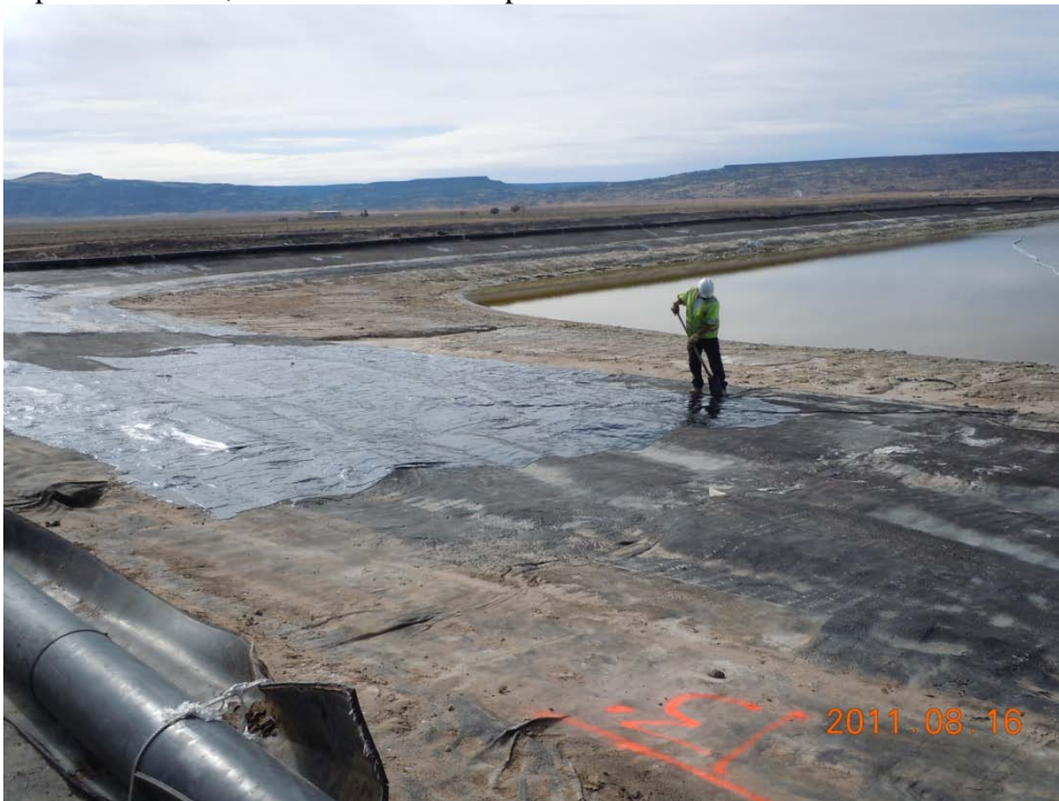
NE corner Evap Pond No. 1, reapplication of Deery Oil top layer over weathered areas.
