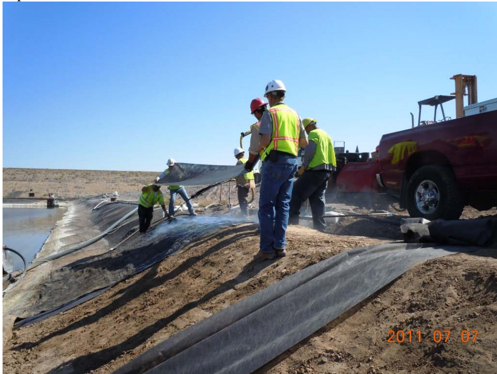
Adding fabric and Deery Oil to extend liner system at top
