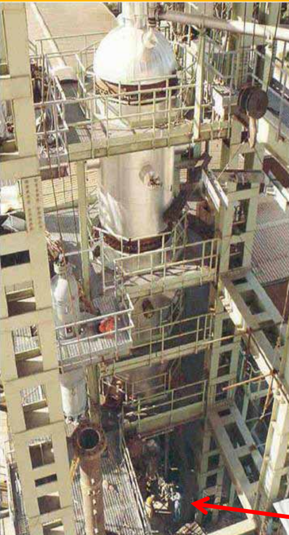
GEST test facility at SIET, reproduced with permission
