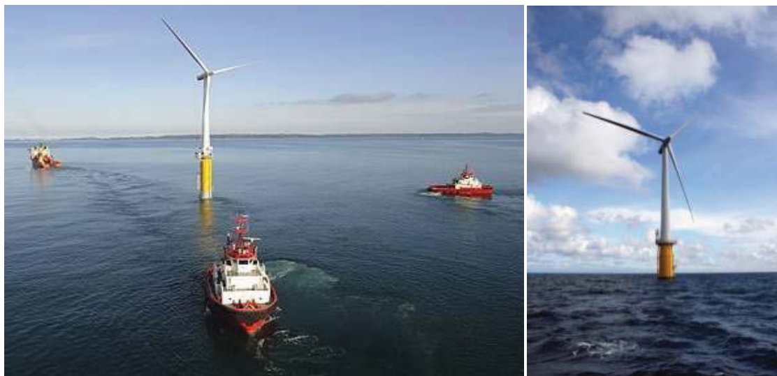
Figure 5-9. First operating deepwater floating wind turbine: Statoil Hywind 2.3-MW prototype during load-out (left) and installed on station (right) (Photos courtesy of Statoil)
