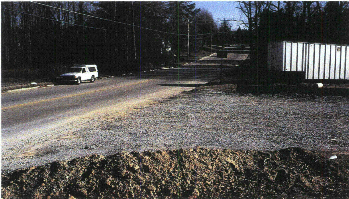
Construction entrance/exit provides an immediate buffer for on-site deposition of mud and sediment.
