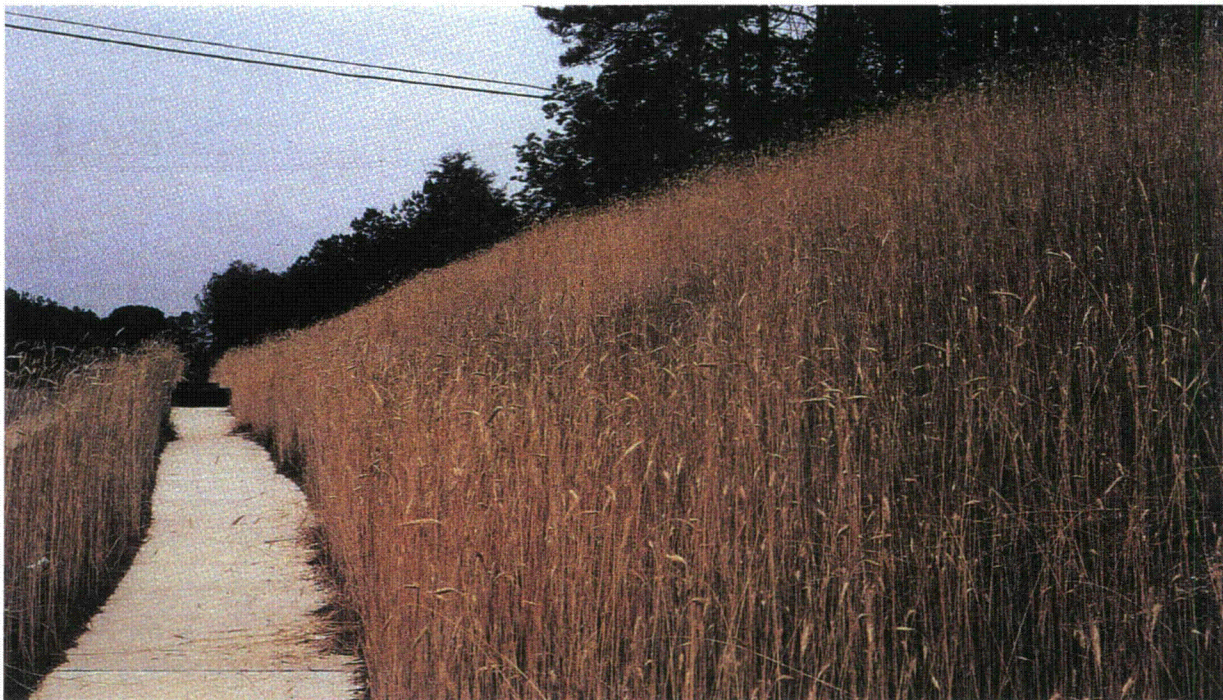
Seeding of temporary vegetative cover provides quick, effective erosion control.
