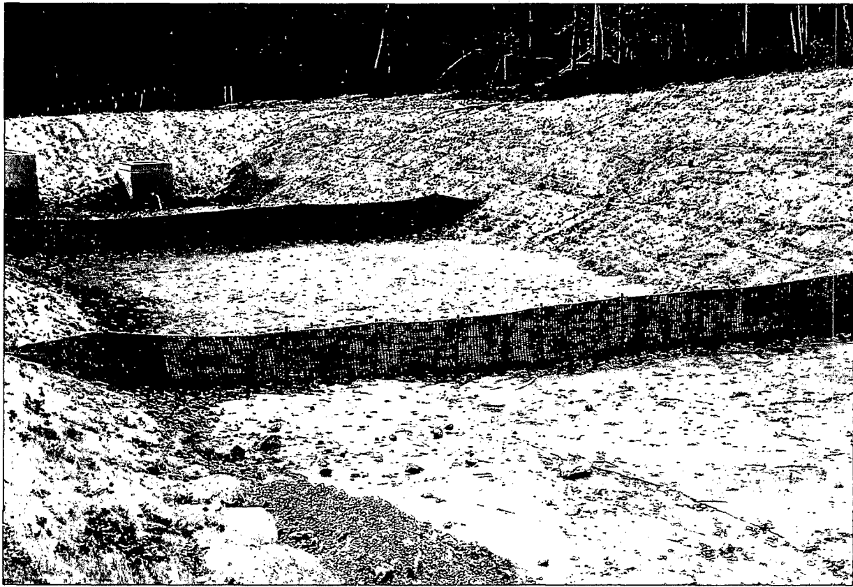
Figure 6.65d Example of porous baffles made of 700 g/m 2 coir erosion blanket as viewed from the inlet.
