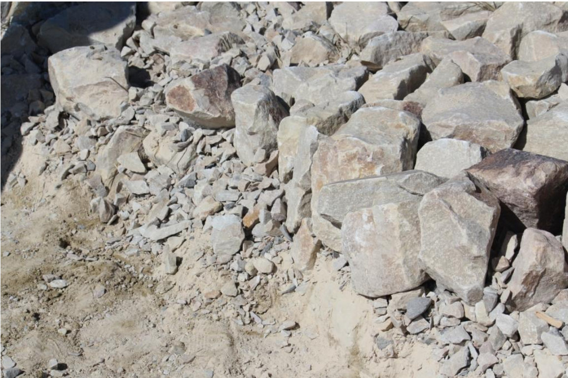
Bottom of test trench showing results of bedding layer emplacement using vibration method
