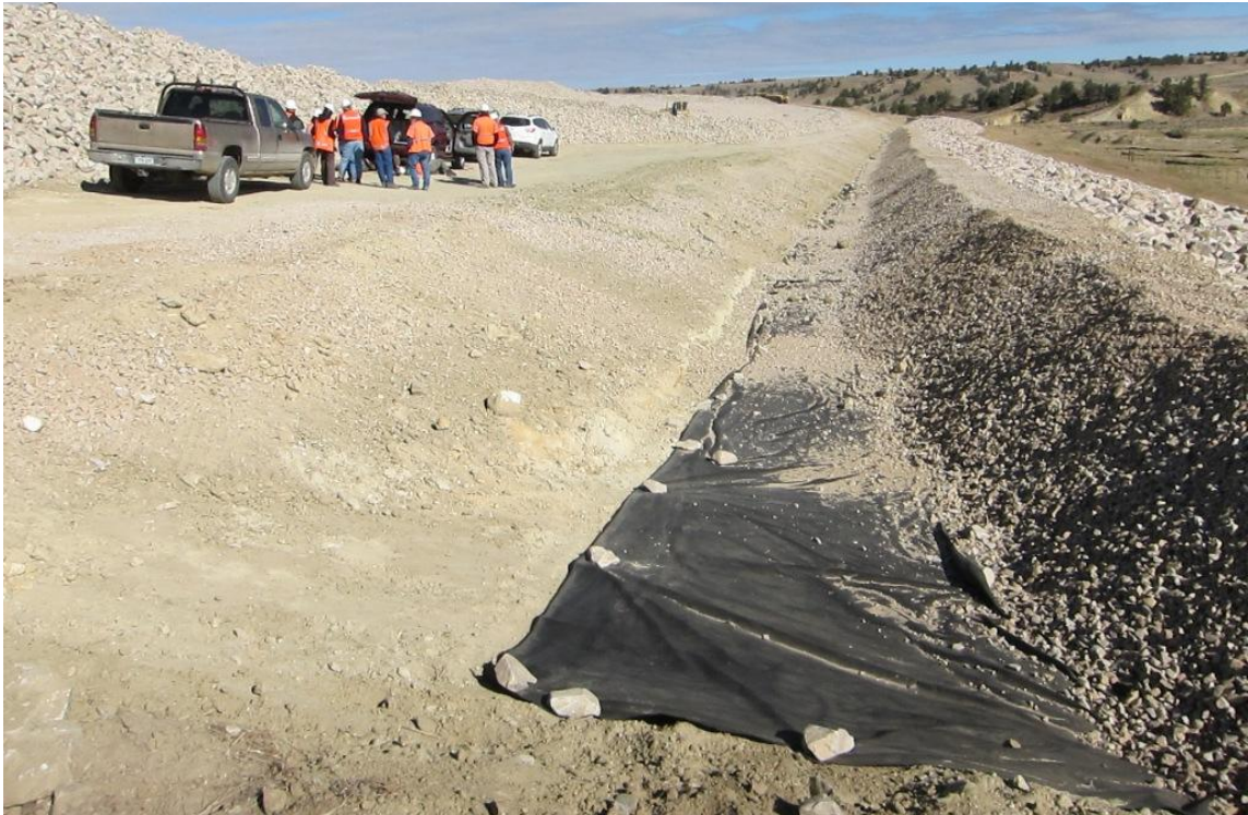
Repair of launch rock structure
