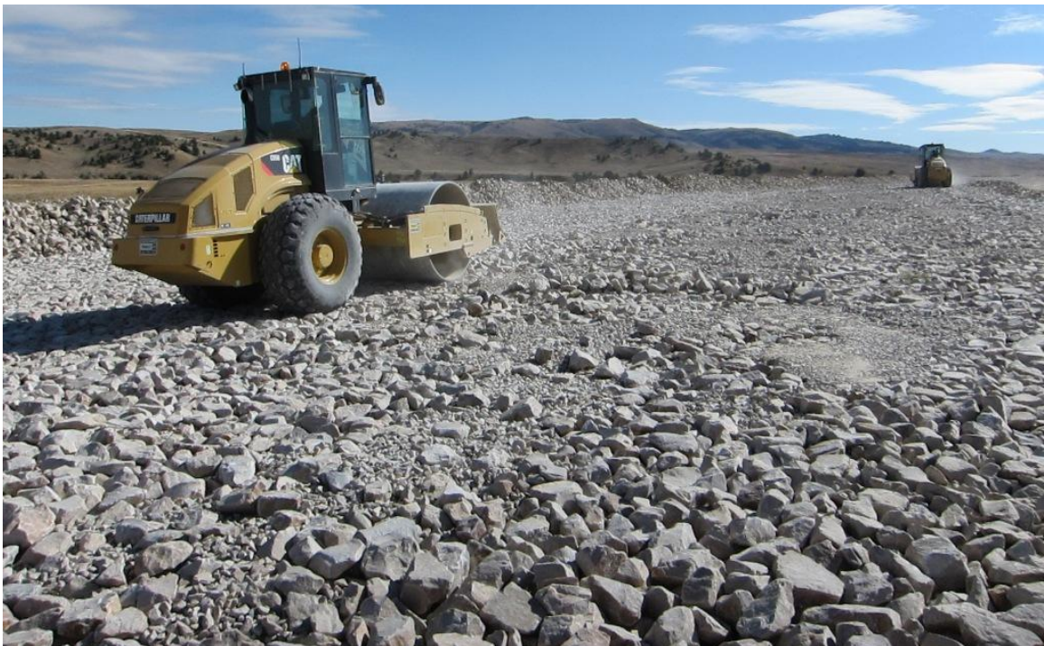
Mechanical vibrators in operation to “shake” bedding layer material under Type C rock
