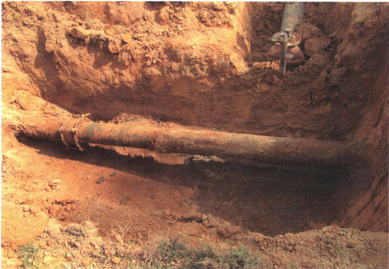
FP Piping to the North Anna Nuclear Information Center (Pipe in the top right corner is for North Anna 3 Site Separation)
