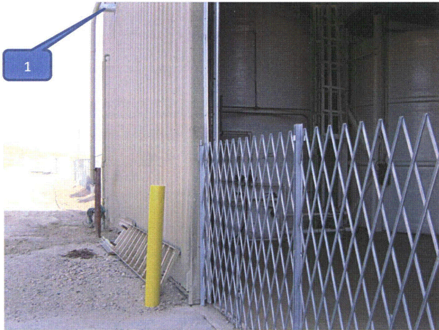
Photo No. 1 Looking northwest at southwest plant door with brine tank partially visible at center. The brine tank's outside vent is indicated by arrow.
