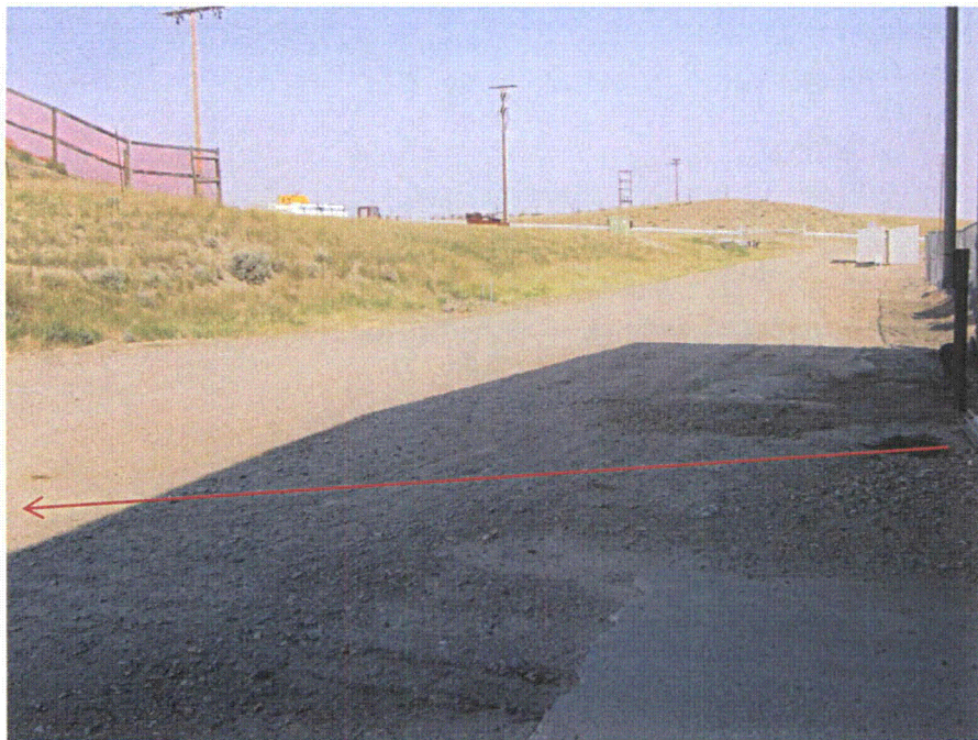
Photo No. 2 Looking northwest at area outside southwest plant door with route of buried culvert shown approximately by line and arrow. The leaking brine flowed through this culvert.
