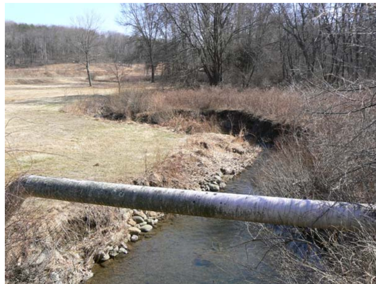
Photo 3. Bank erosion on Walker Run immediately south of the Market Street Bridge
