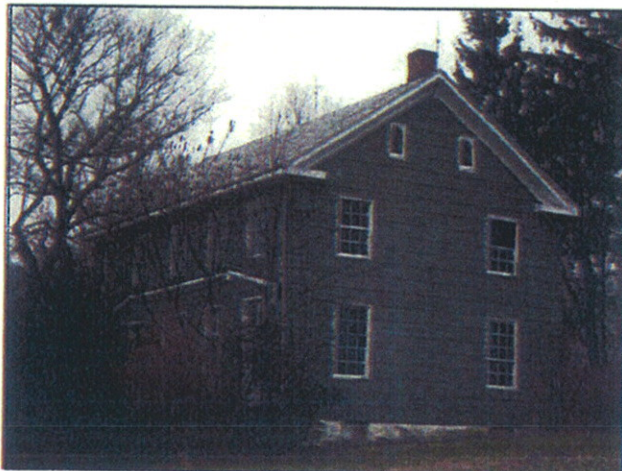
GAI-14 (155061) – House, 49 Bell Bend Road, Salem Twp. (Recommended Not Eligible)
