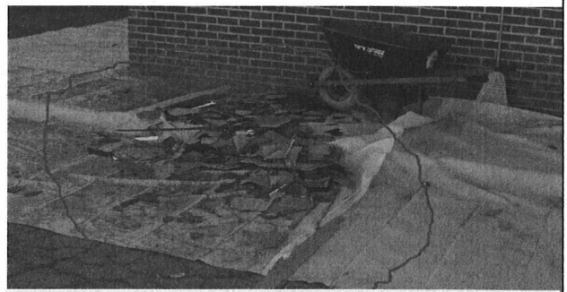
Public health hazard due to the improper demolition and handling of asbestos containing shingles
