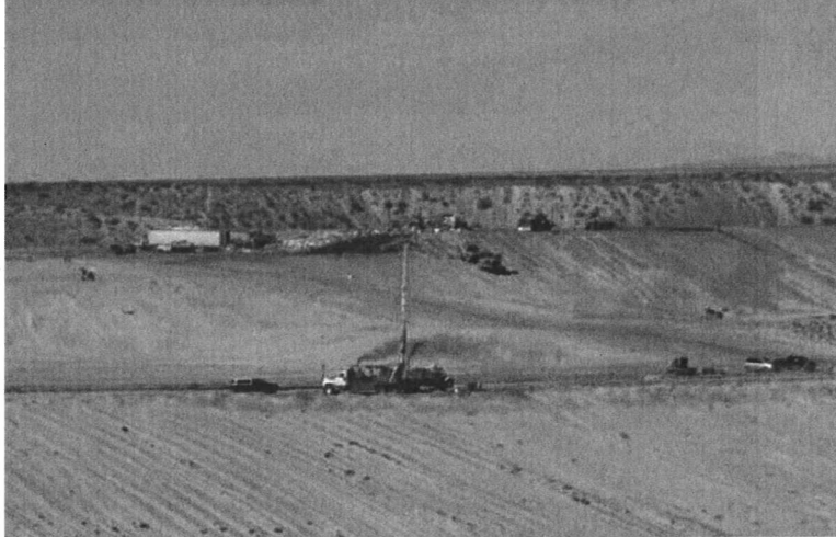
Camino Real Landfill— Installation of a methane gas monitoring well
