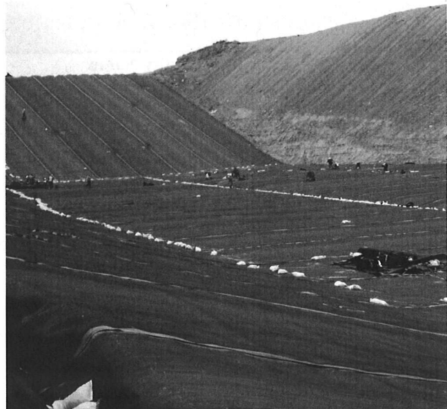
Installation of the protective liner and leachate collection system at the Rio Rancho Landfill
