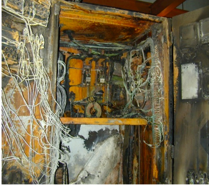
Figure 10: Combustible components within the switchgear
