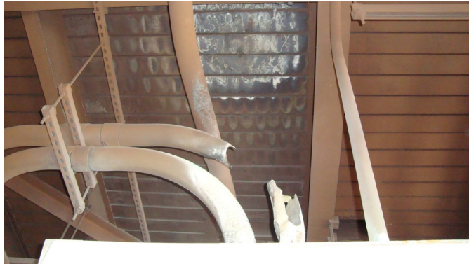
Figure 1: Photo of the conduit damage above a switchgear
