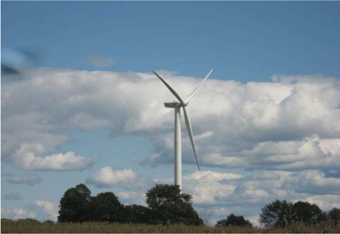
Stoney Corners, Missaukee County – 2 – 2.5 MW, 2008
