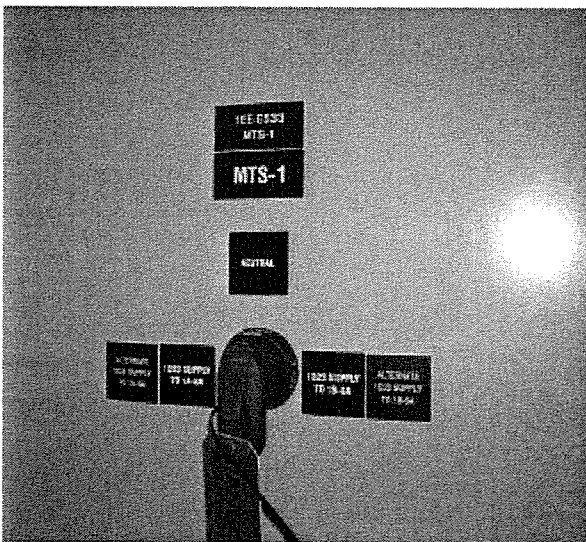
Figure 2: Alternate Supply Manual Transfer Switch for
