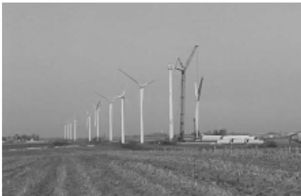
Figure 6. A large crane is used to raise a rotor into position. Photo courtesy of AWEA.
