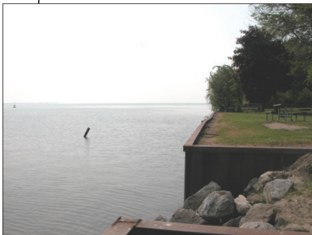
Figure 1. Lake Erie shoreline hardening with steel sheet piling (Photo credit: Greg Norwood).
