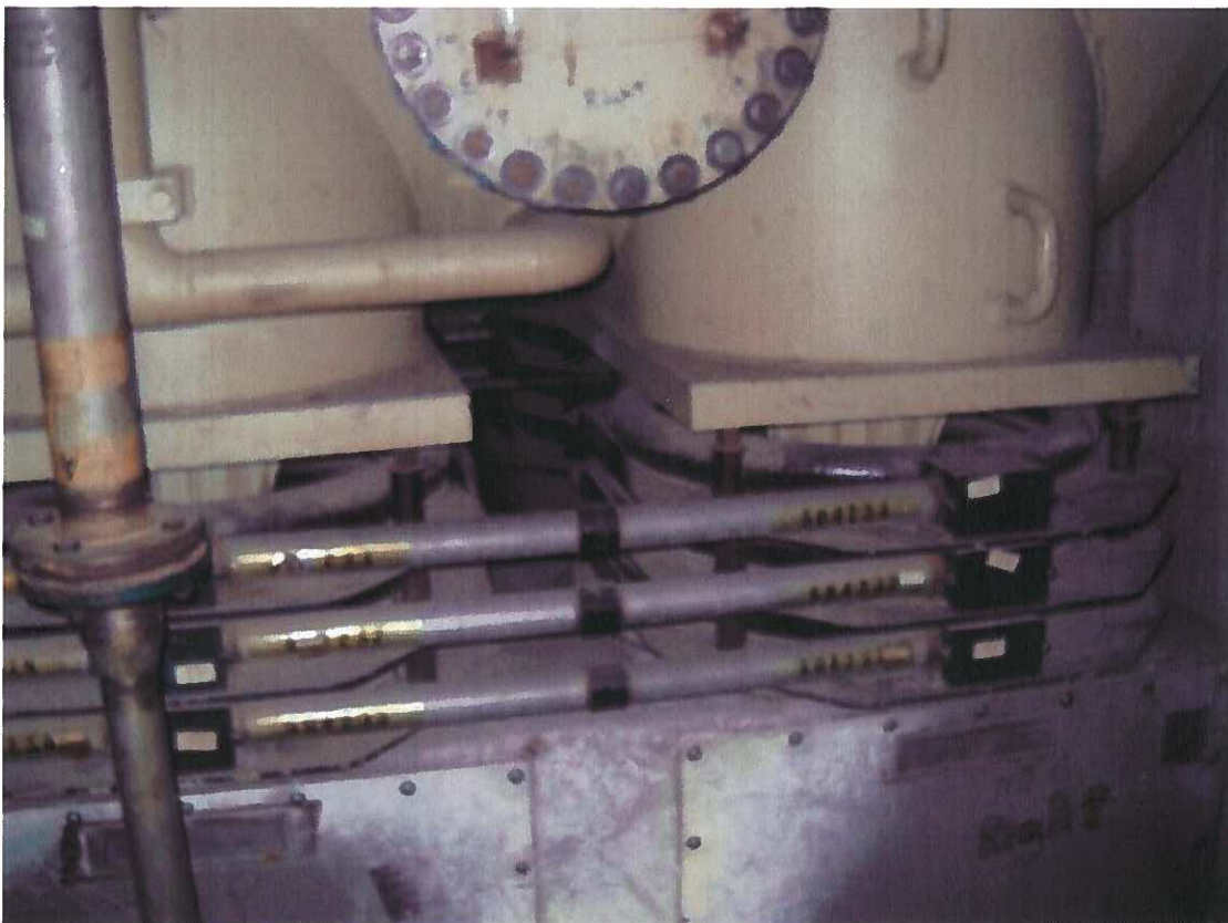
Figure X-1- Typical Configuration of Main Generator CTs
