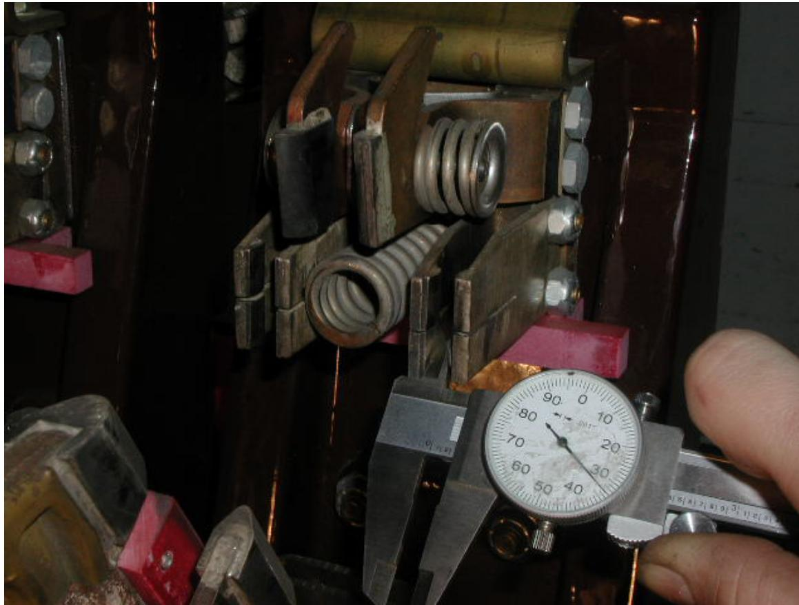
**VERIFY the moving main and arcing contacts are approximately centered in the stationary contacts**
