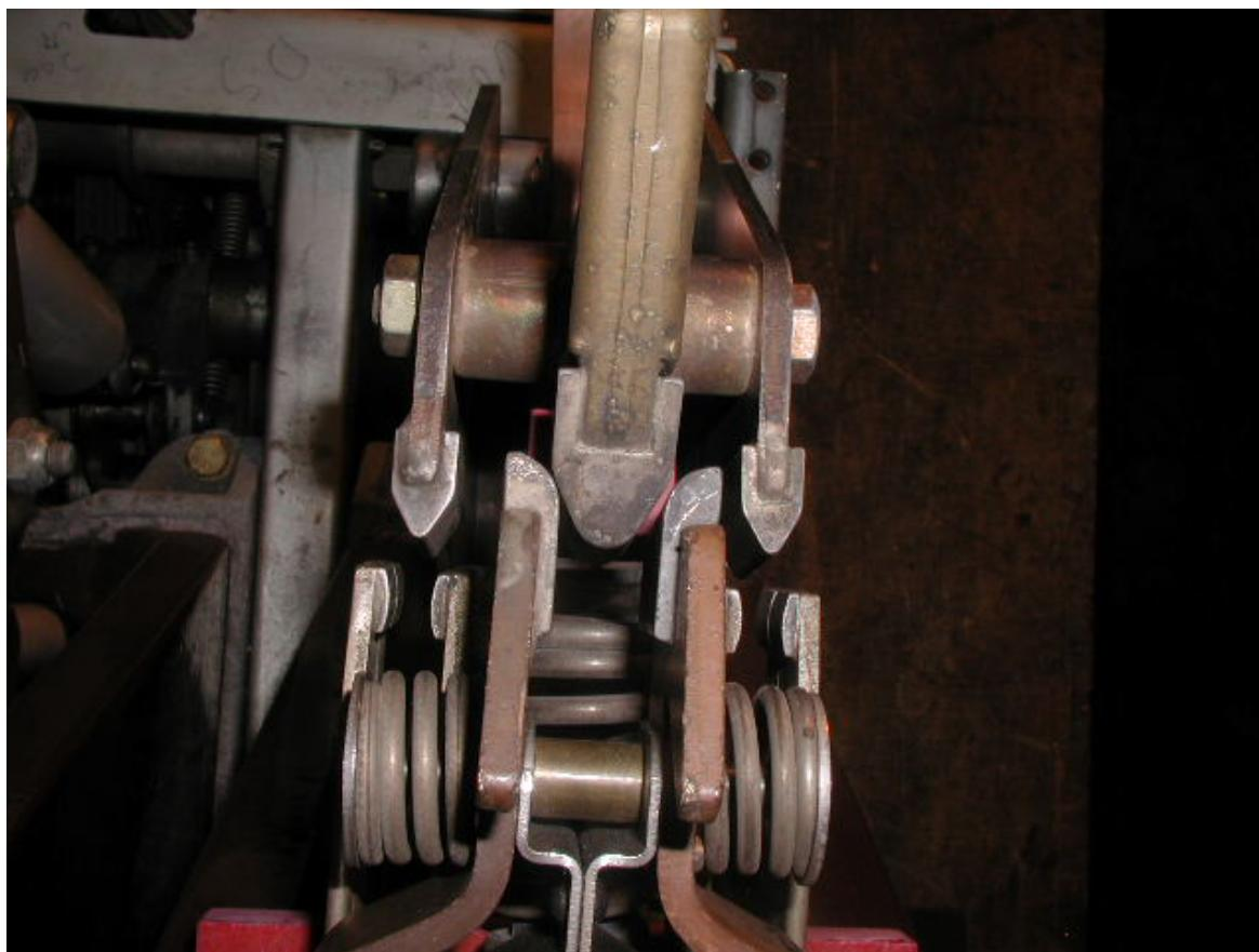
**When the arcing contacts just touch , verify the main contacts must have a minimum 0.0625" gap between the stationary and moving contacts**
