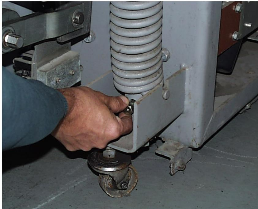
**CONTINUE to charge the breaker until the first arcing contact touches, Measure the contact gap of this phase.**
