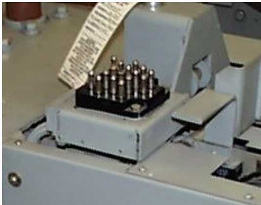
New 4160 VAC Vacuum breaker (back view)
