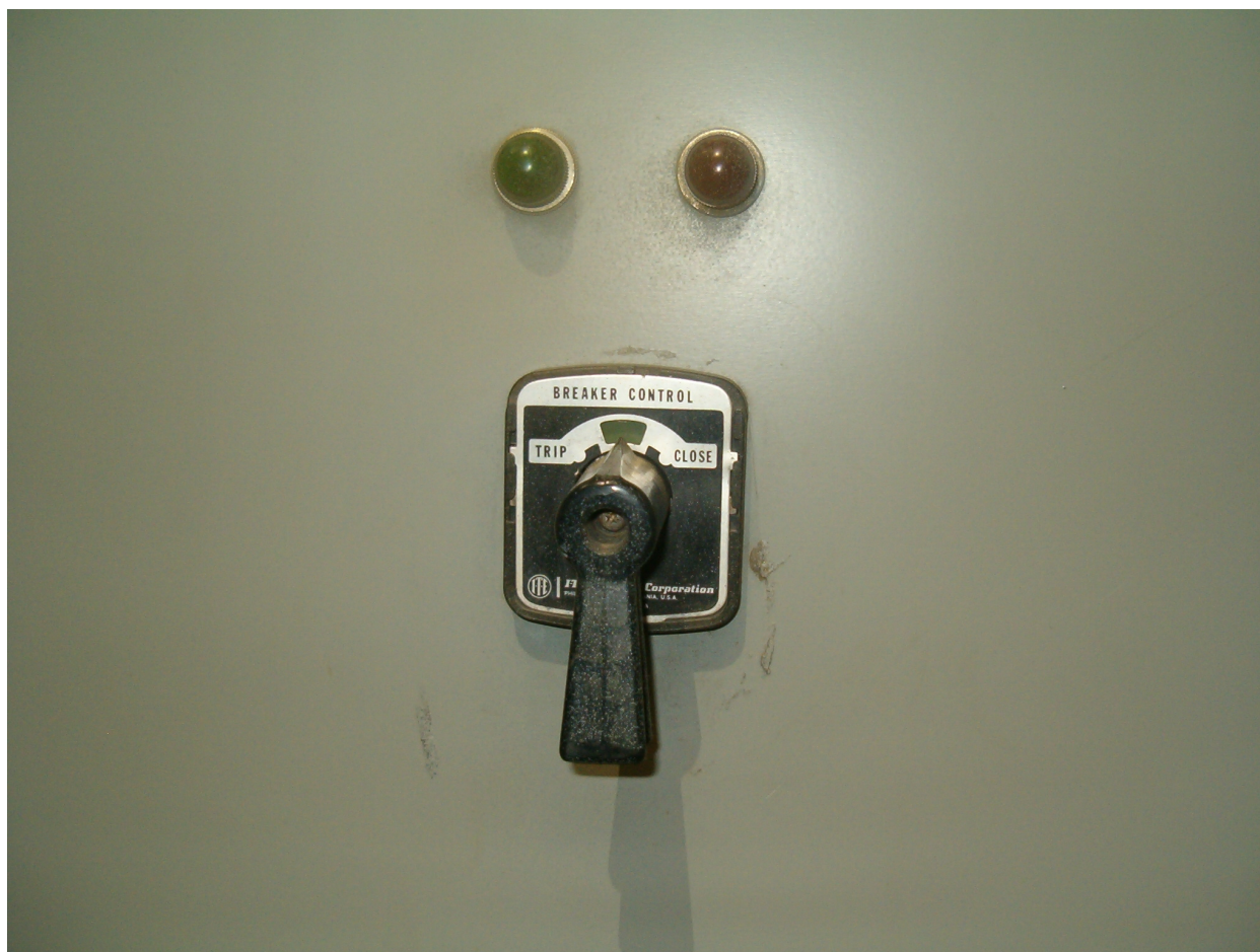
FIGURE 3-1 Cubicle breaker control switch
