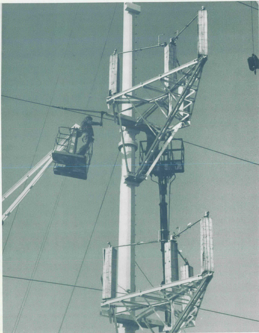
SKYHIGH —The second of three switches is attached to the 110-foot steel pole in the new Hampton 161-kV line.
