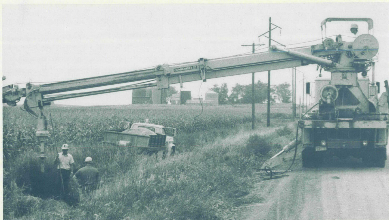
CONSTRUCTION —Corn Belt crews build the Lakota Tap, a 2.5 mile stretch of 69-kV line located in northern Kossuth County. Corn Belt personnel were responsible for a significant amount of construction in 1986.
