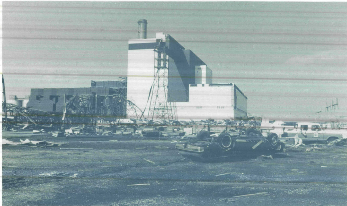
AFTERMATH —The Neal #4 generating station and its coal handling system were severely damaged by a tornado that hit the facility near Sioux City at 7:50 p.m. Monday, July 28, 1986. Repairs on the 600-megawatt plant are expected to be completed in late spring, 1987.
