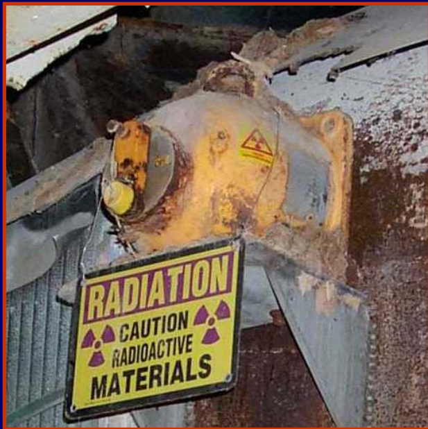
Level gauge mounted on a process tank at a paper mill
