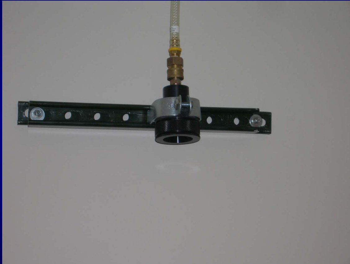
Room air sample head in iodine room
