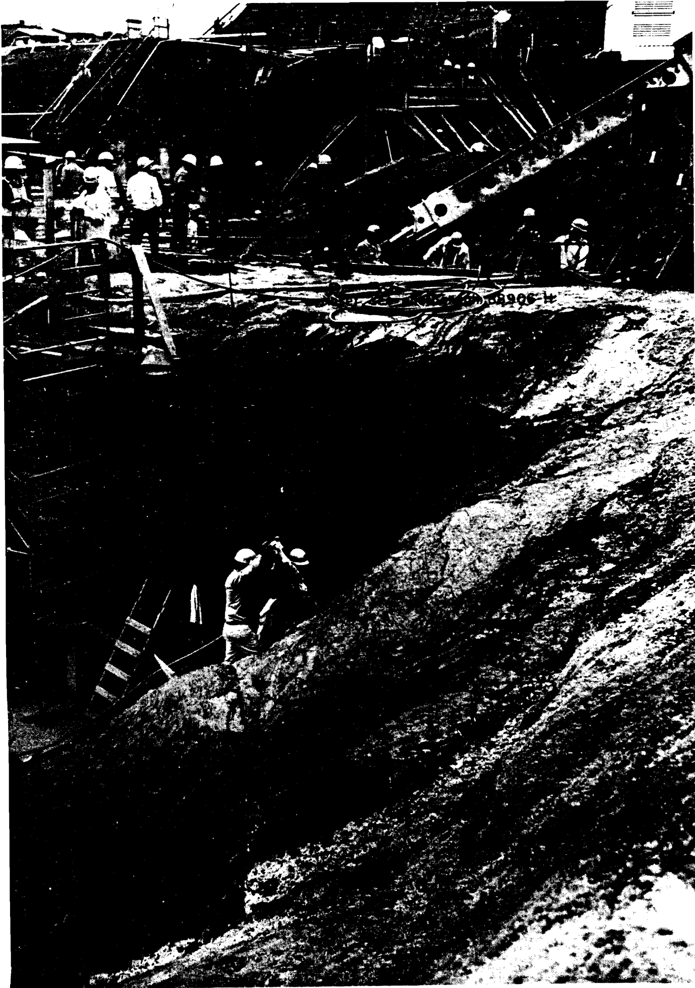
Watts Bar Nuclear Plant Tennessee Valley Authority 88902-F January 16, 1974 Gary W. Krantz, Knoxville Fault shown cutting across Auxiliary Building at A4+28 feet and east-west reactor center-line, through SE perimeter of Reactor #1, and into Auxiliary Building West Wall near U line. Viewed southwest.
