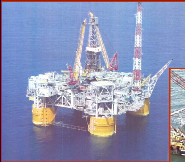
Off Shore Oil Drilling Platform
