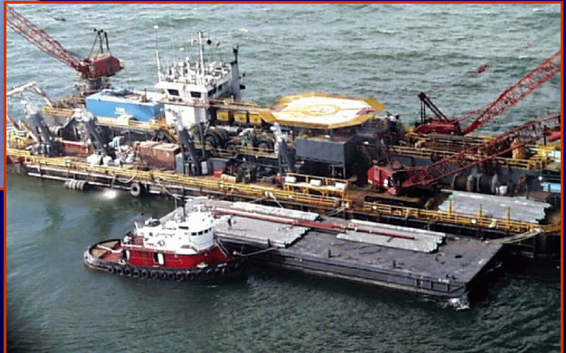
Lay Barge (pipe laying operation)
