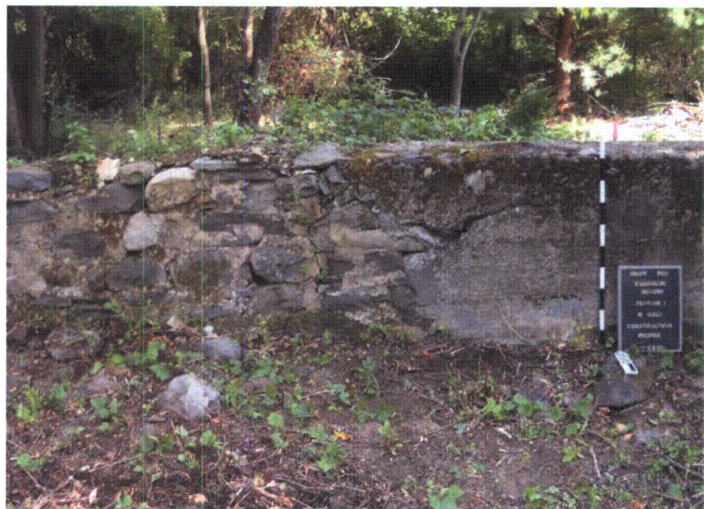
Photograph 14-9. Site 36LU283: Feature 2, North Foundation Wall Detail showing Dovetail of Both Construction Methods, Facing North
