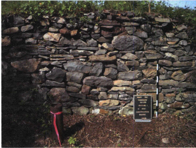
Photograph 14-6. Site 36LU283: Feature 2, Detail of West Foundation Wall Construction, Facing West
