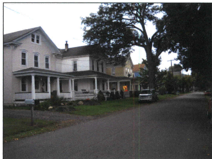
Photograph 20-17. Wapwallopen Historic District, Representative
