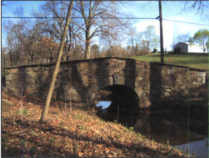
Photograph 20-12. North Market Street Bridge, Facing Southwest
