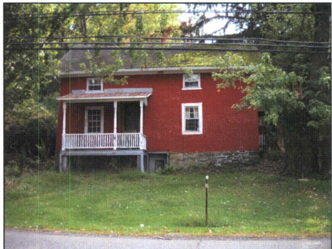
Photograph 20-7. Woodcrest, Secondary Dwelling, Front Elevation, Facing East
