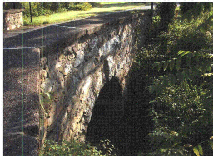
Photograph 6-23. Lot 4, Stone Arch Bridge (155054/GAI-06), Facing Northeast
