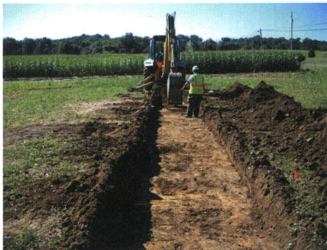
Photograph 10-6. Site 36LU279: Trench Excavation in Progress.
