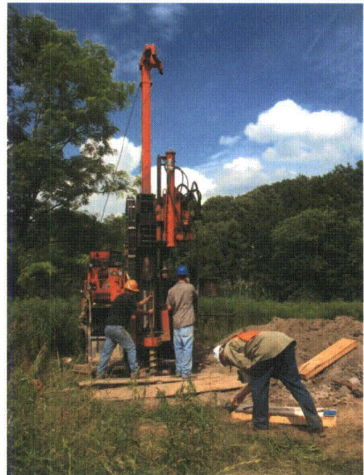
Photograph 6-12. Deep Testing in Area 6, Section 1, showing Drill Rig Excavating a Soil Coring in Base of Trench, Facing North
