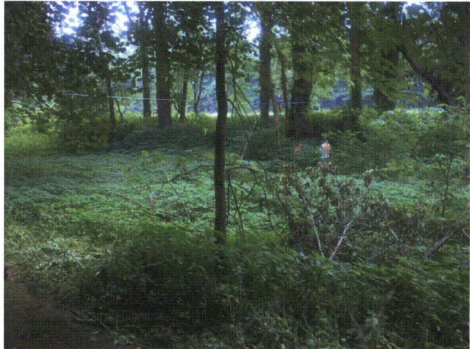
Photograph 6-15. View of North Branch Pennsylvania Canal in Area 7 showing Dry Canal Prism, Facing Southwest
