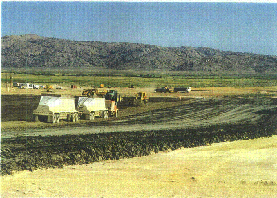
Photo 11 - Area 3A - Placing Radon Barrier, 1994
