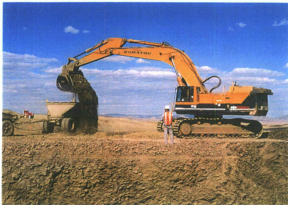
Photo 8 - Loading Cody Shale for haulage to tailing area
