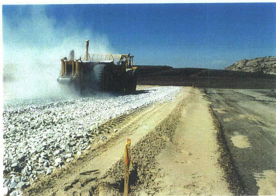
Photo 33 - Area 2A - Laying 2" mulch, May 4, 1995
