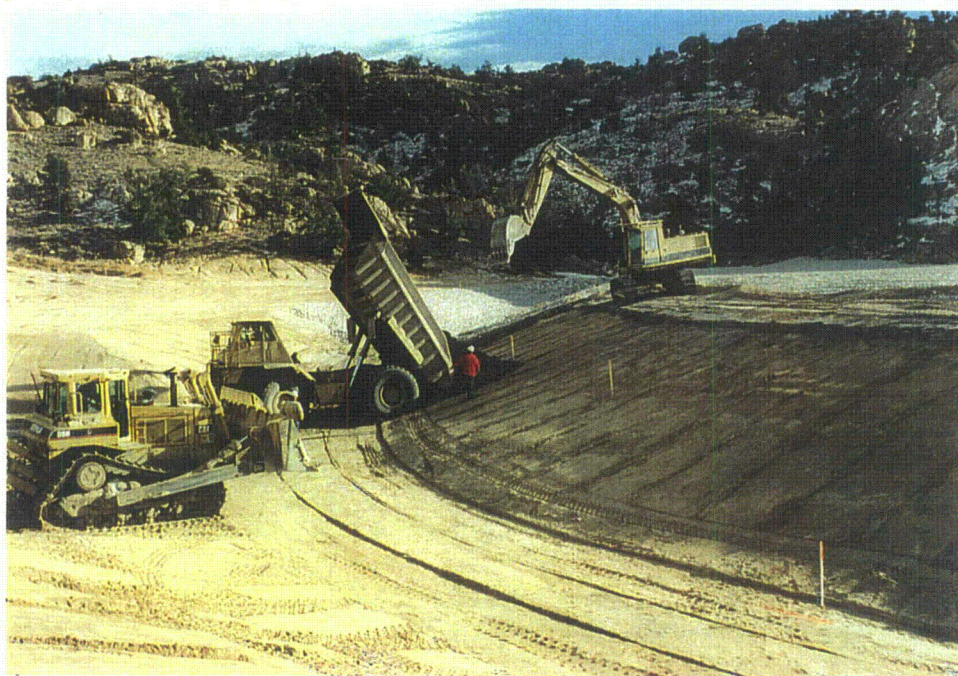
Photo 25 - North Diversion Ditch by confluence, November, 1997
