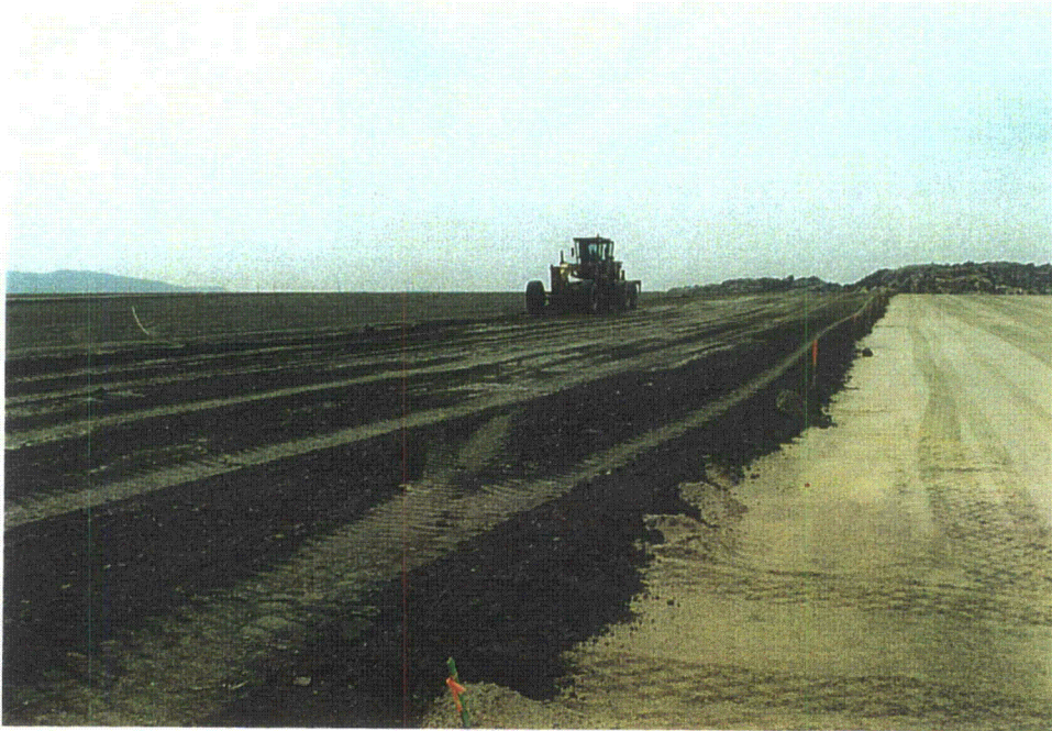
Photo 10 - Area 1B - sacrificial clay placement / spreading to 4", May, 1996
