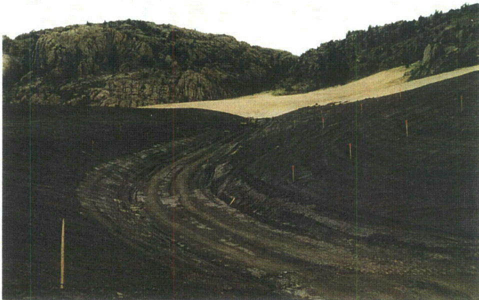
Photo 28 - Area 1B – South Diversion Ditch - Clay layer, July, 1996
