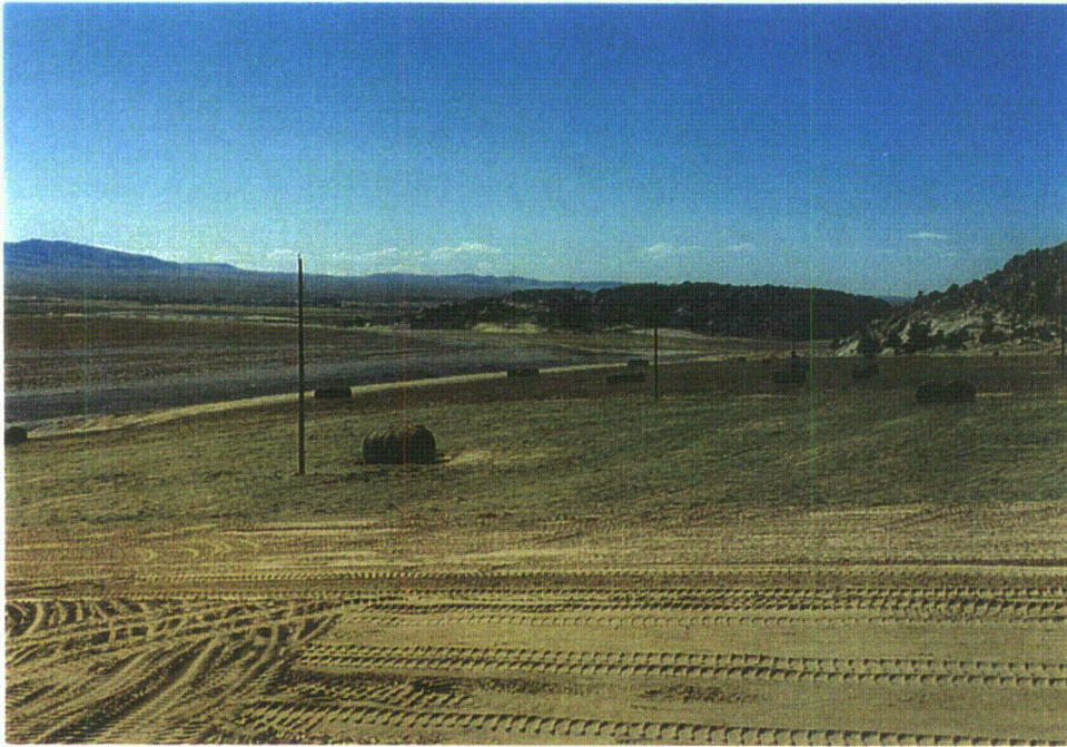
Photo 43 – First layer of hay mulch for reseeding in North East Borrow Area – October, 1998
