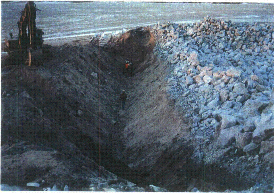
Photo 39 - South Diversion Ditch - measuring scour trench, December, 1997
