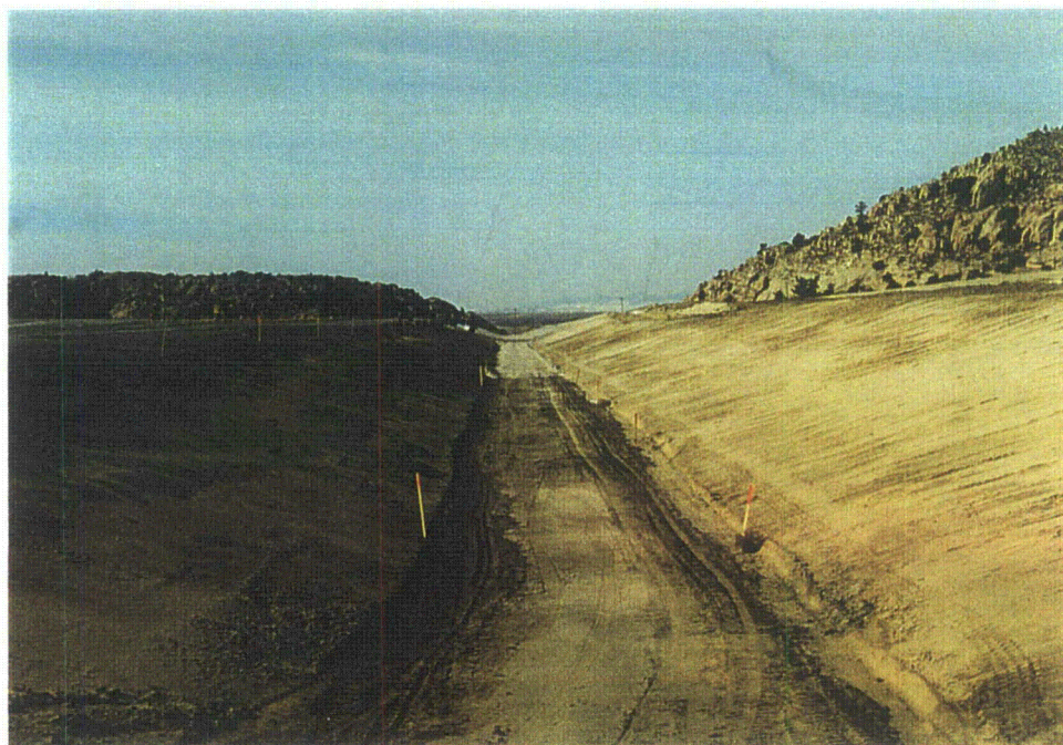
Photo 24 – North Diversion Ditch - Placement on inside slope, October, 1997
