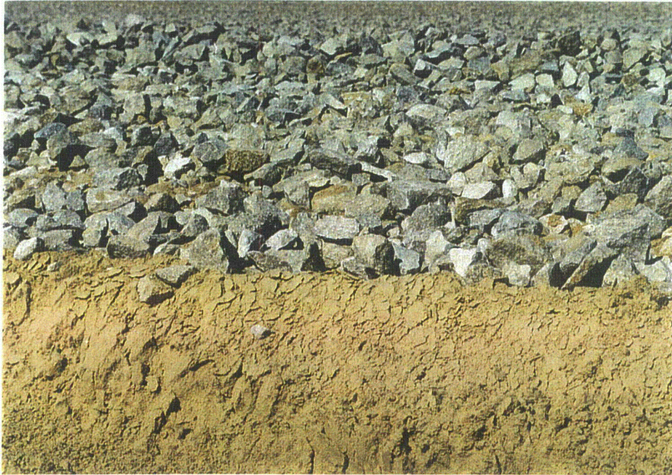
Photo 34 - Area 3A/3B - 4" D_{50} 2" rock mulch over top of 10" - 12" Borrow soil, 1994
