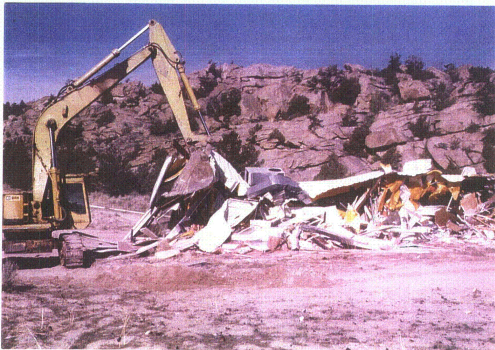
Photo 2 - Office Demolition, May 13, 1997
