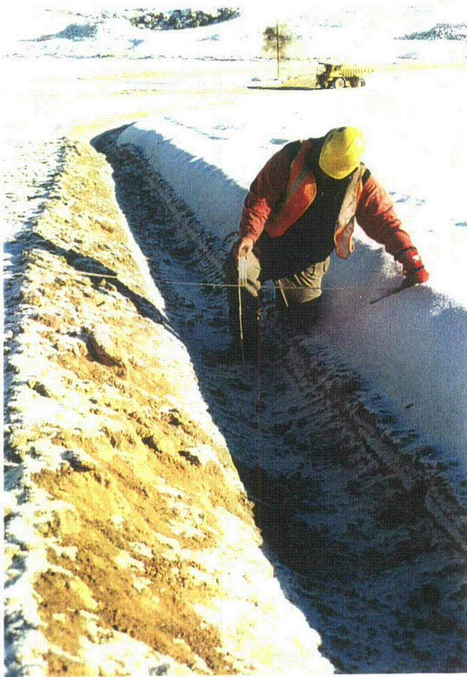
Photo 38 - Key Trench by Area 3A - depth measurement, December, 1997
