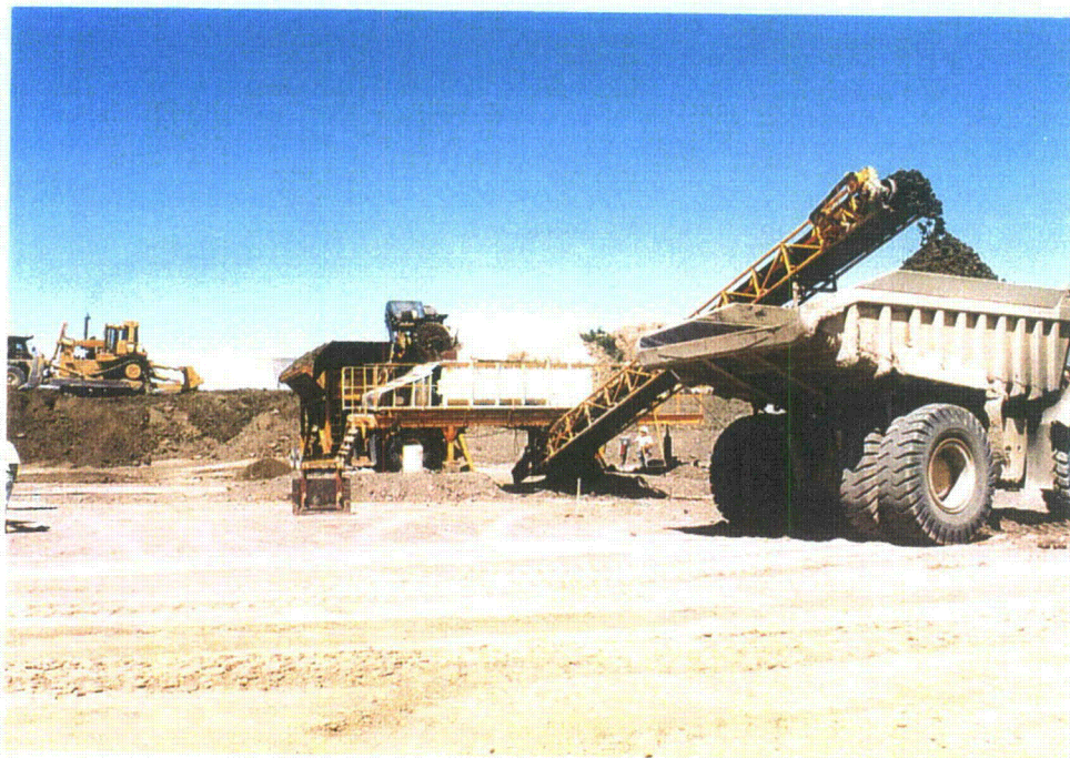
Photo 16 - Area 2A - Pug Mill moisturizing clay, August, 1995
