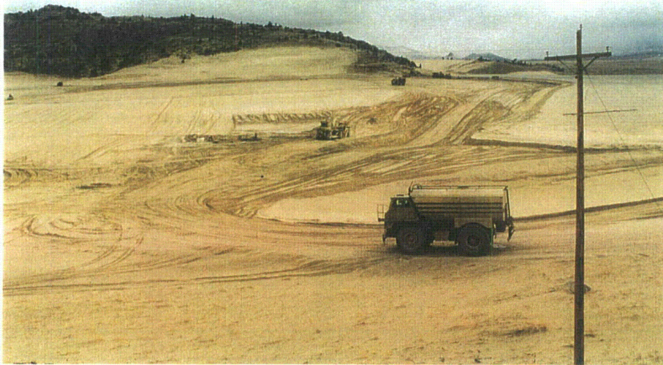
Photo 4 - Area 1B Right - Preparing subgrade, April, 1996
