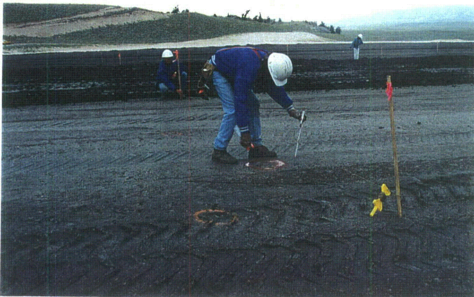
Photo 19 - Area 2A - Checking Grade and Thickness, August, 1995
