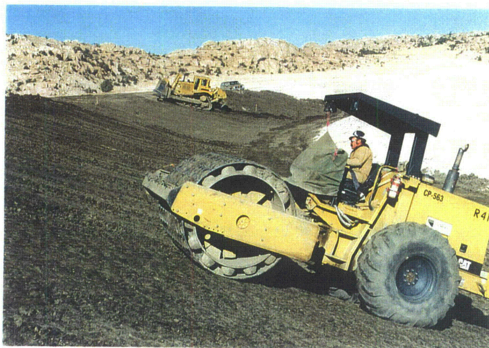
Photo 27 - Compacting Radon barrier South Diversion Ditch, October, 1995
