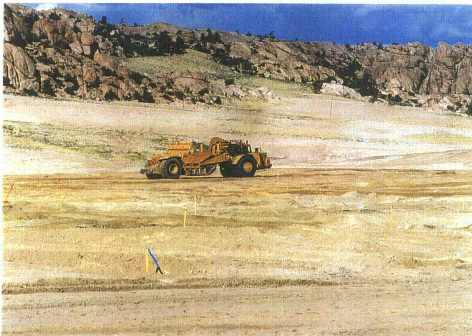
Photo 5 - Area 3A - Shaping subgrade, 1994
