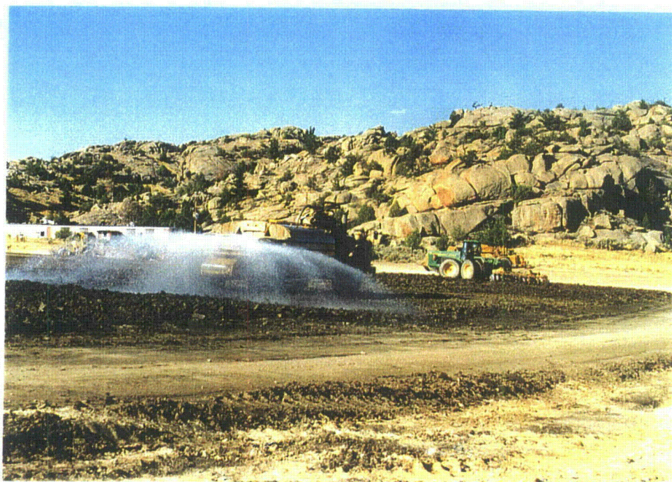
Photo 17 - Area 3A - Moisture conditioning stockpiled clay, 1994
