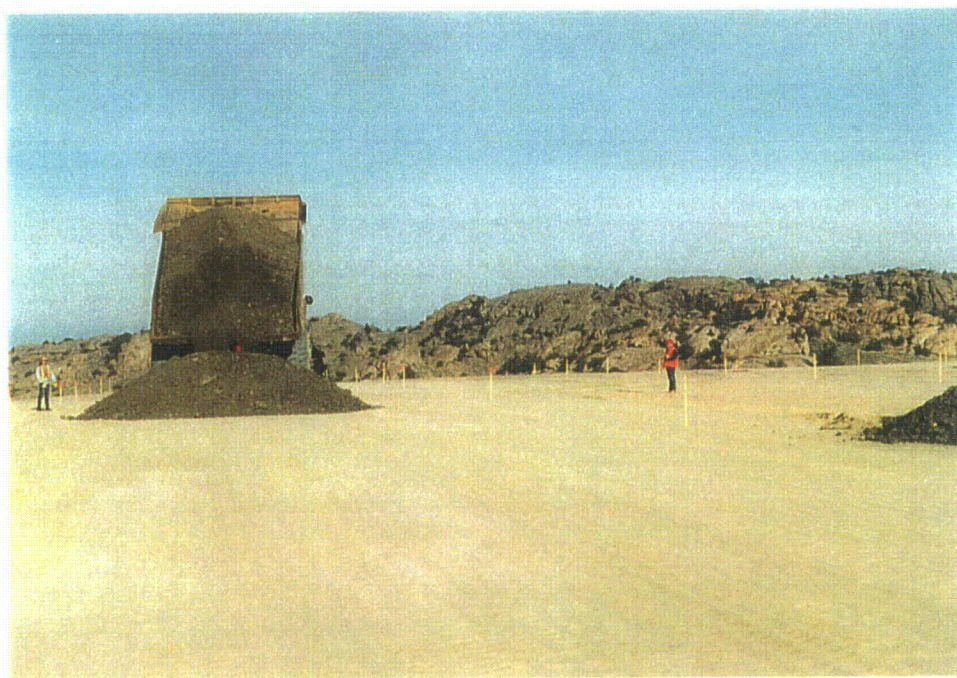
Photo 9 - Area 1B - Sacrificial clay placement, July, 1996
