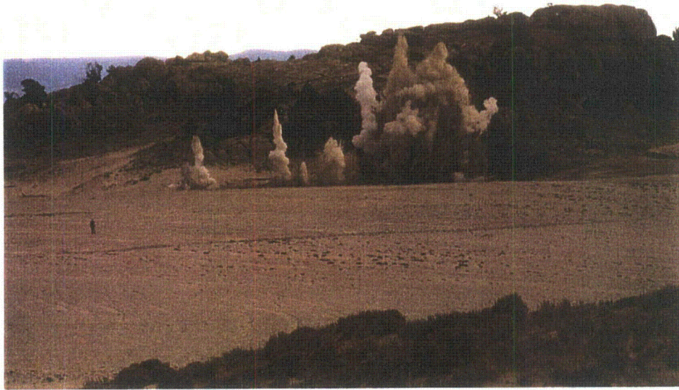
Photo 22 - Northeast Diversion Ditch - Blasting, 1995
