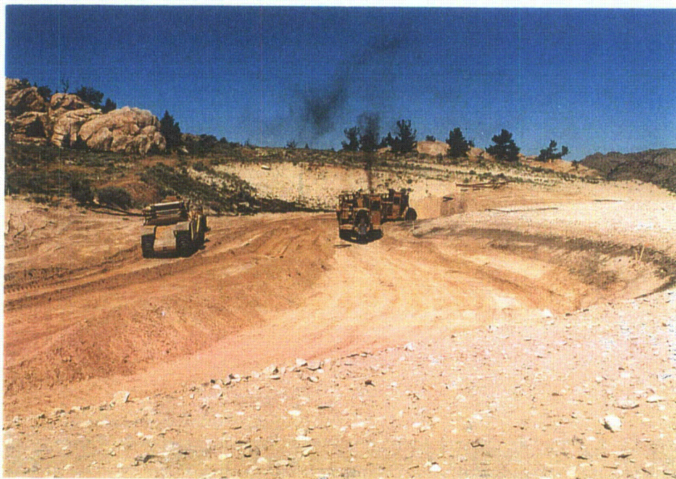
Photo 26 - Excavating and shaping South Central Diversion Ditch, August, 1995
