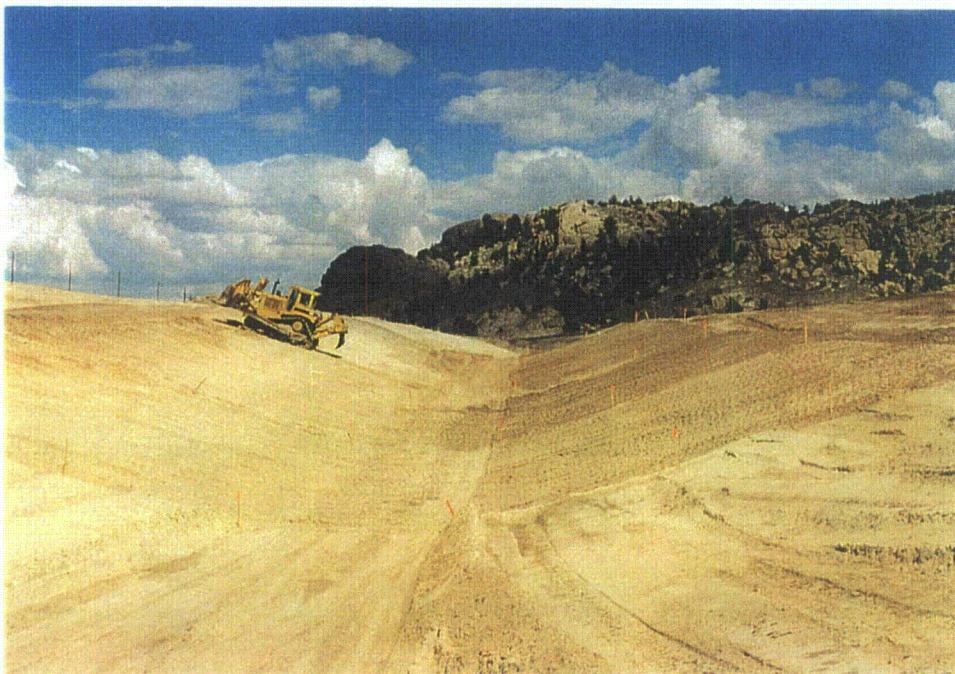
Photo 23 - North Diversion Ditch - Compacting subgrade, July, 1997
