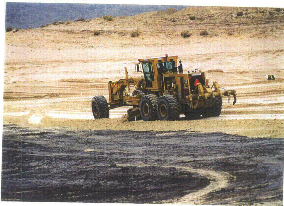
Photo 21 - Area 3A - Spreading borrow soil layer, 1994
